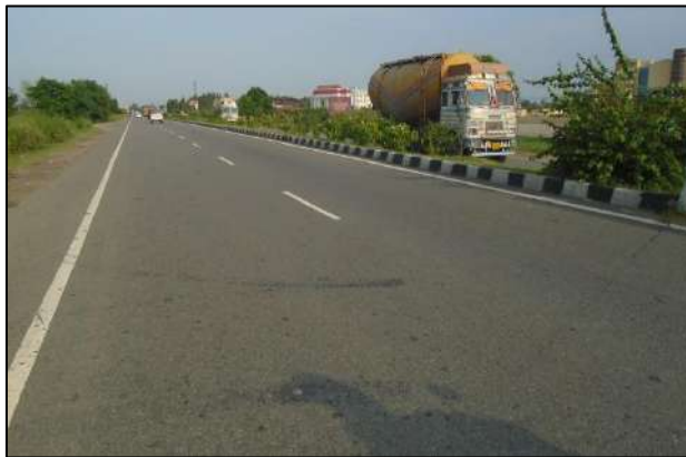
Pavement Condition at km. 6+950
