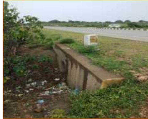
HPC at km. 380+328 (RHS)
