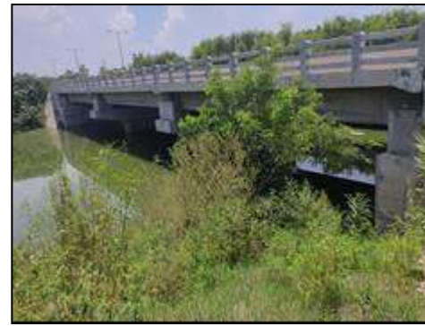
Minor Bridge at km 59+237 (New Structure View)
