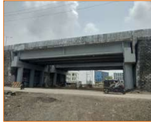
Side View of VUP at km. 58+570 (LHS)
