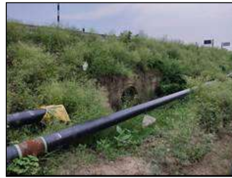
HP Culvert at km. 1+135
