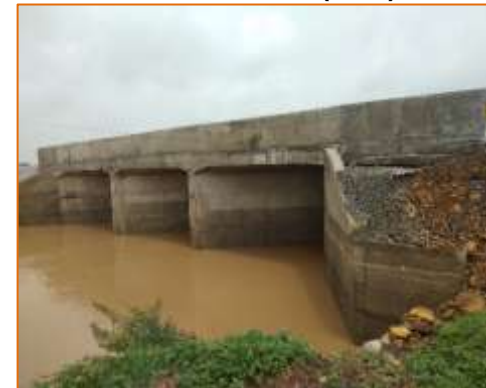
Side View of Minor Bridge at km. 21+955 (LHS)
