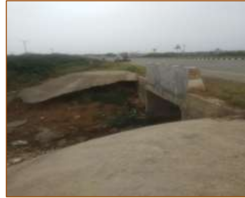
Slab culvert at km. 441+648 (LHS)
