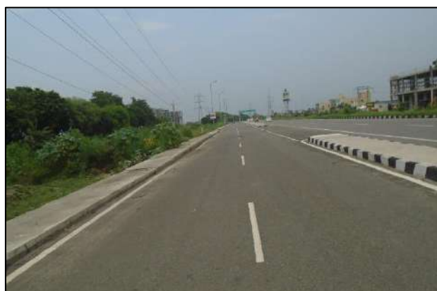
Service Road at km. 0+630 (LHS)
