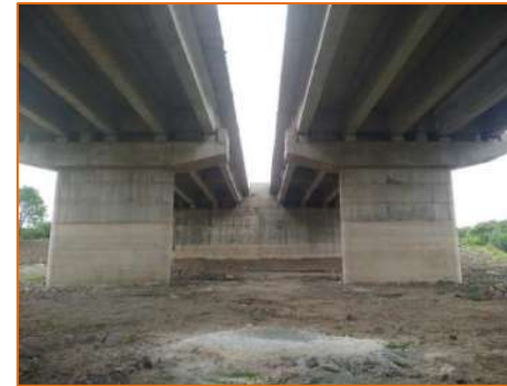
New Major Bridge at km. 298.190
