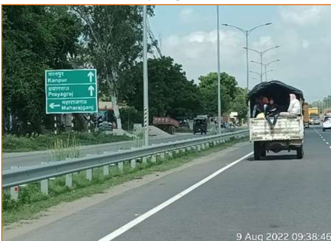
Sign Board at km. 767+100.
