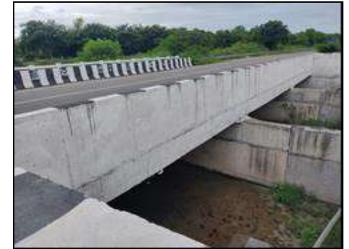
Minor Bridge at km. 72+900 (Top View)
