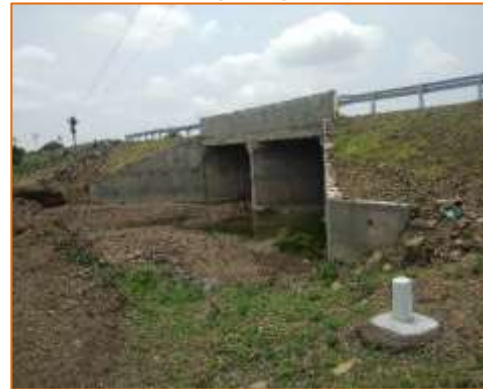
Side View of Minor Bridge at km. 64+660 (RHS)
