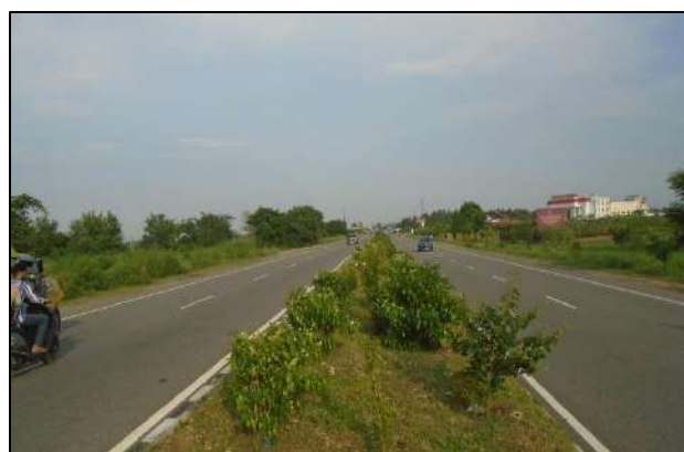
Median Plantation on project highway
