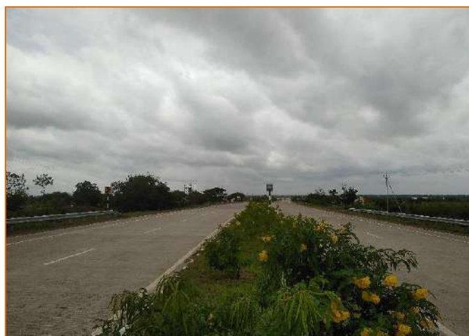
Median Plantation at km. 313+450
