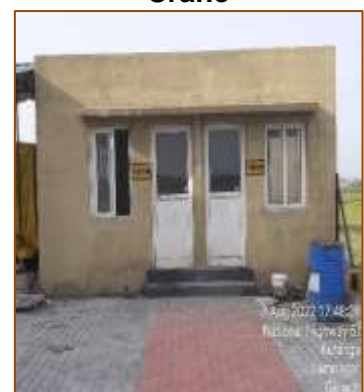
Panel / Pump Room
