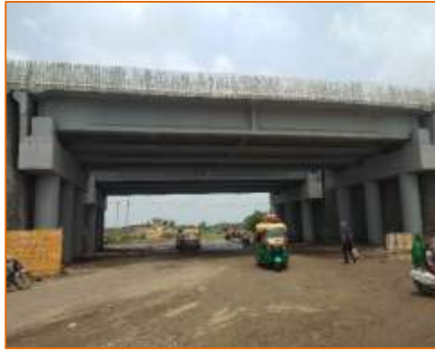
Side View of VUP at km. 57+975 (RHS)
