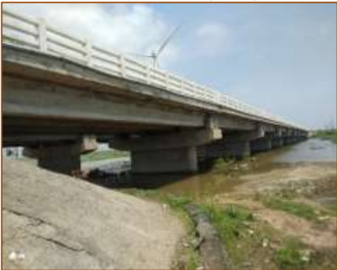
Side View of Major Bridge at km. 415+929 (LHS)
