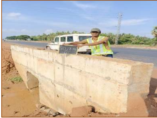
Box Culvert at km. 30+874
