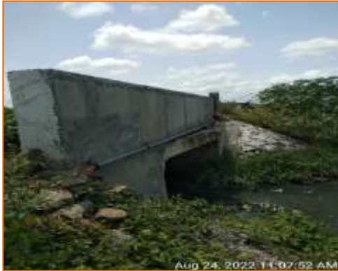
Box culvert at km. 101.823 - LHS (New Construction)
