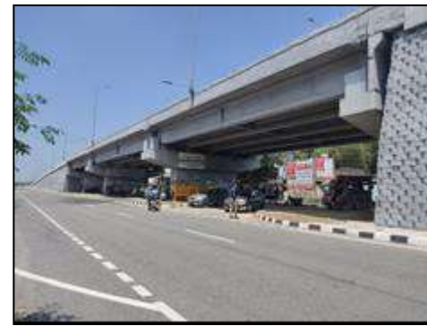
Flyover at km. 59+818
