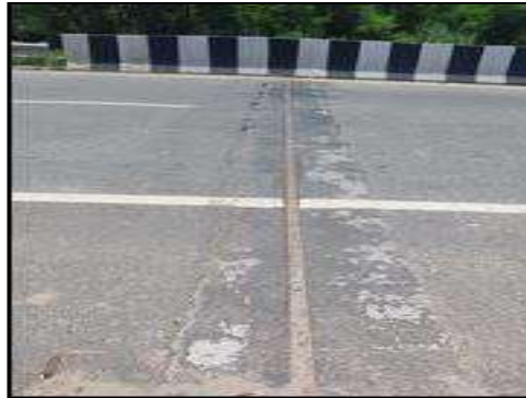
Minor Bridge at km 59+237 (Expansion Joint)
