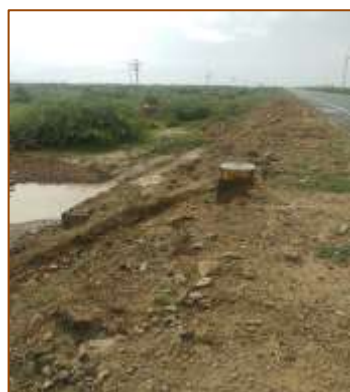
MJB at km. 487+054 (RHS)
