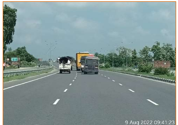
Road Marking at km. 761+200.
