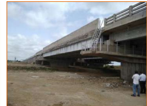
Rail Over Bridge at km. 294.125
