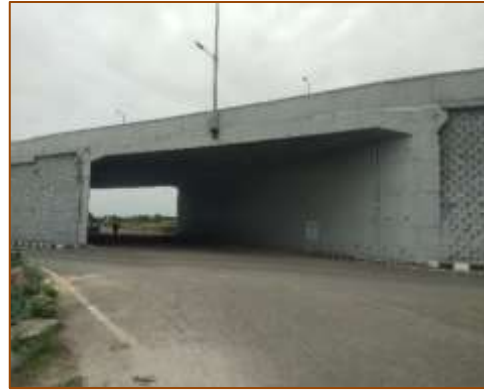
VUP at km. 397+096 (RHS)
