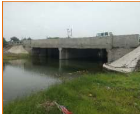
Side View of Minor Bridge at km. 67+865 (LHS)
