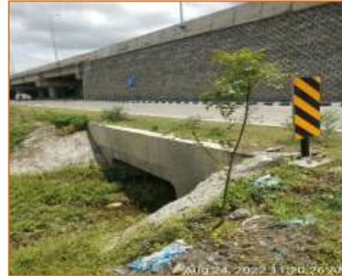
Box culvert at km. 102.650 - LHS (MCW & SR - New Construction)
