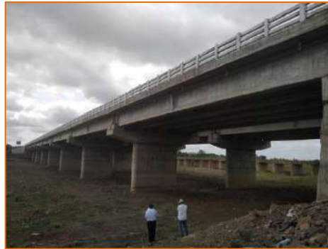
New Major Bridge at km. 298.190
