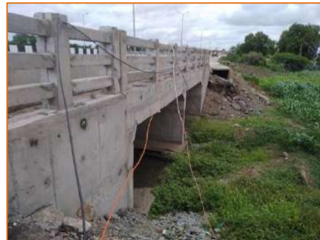
Reconstruction of Minor Bridge at km. 284.835
