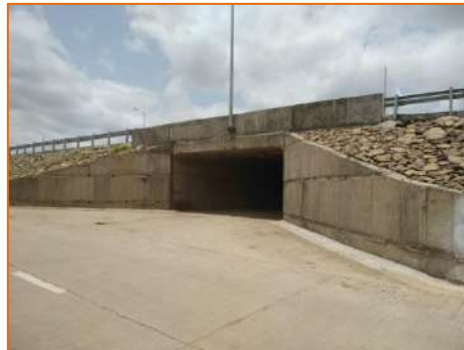
Pedestrian Underpass at km. 284.500
