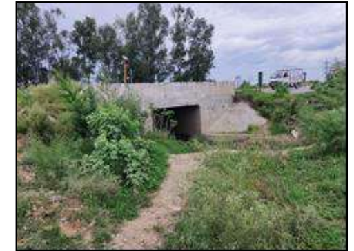
Box Culvert at km. 10+481
