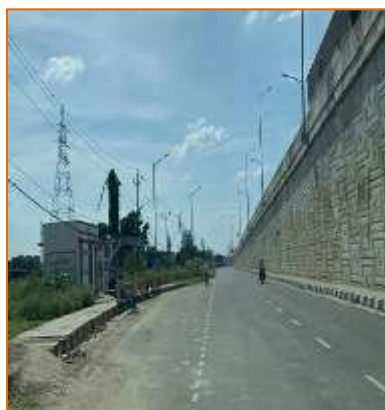
Service Road at km. 781+450
