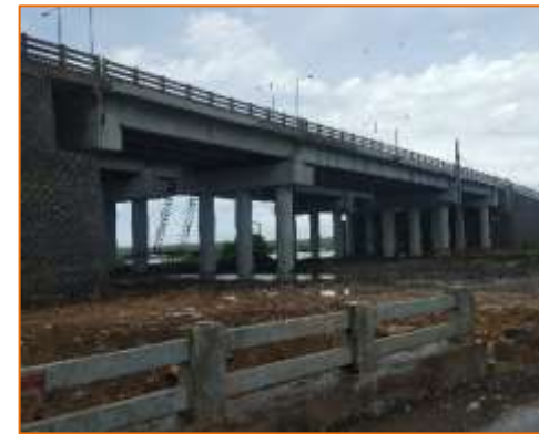
Side View of ROB at km. 0+527 (RHS)
