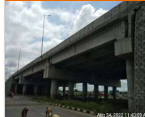
Side View of Flyover at km. 103.801 (RHS)
