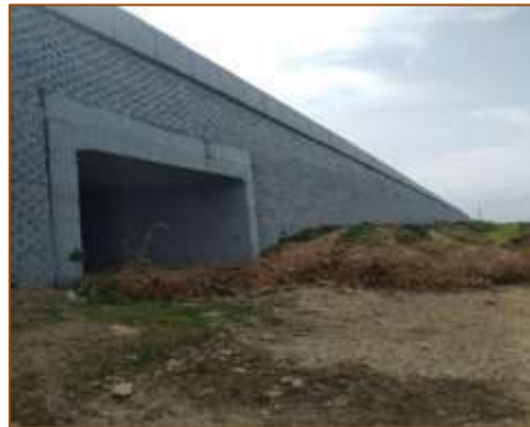
VUP at km. 393+695 (RHS)
