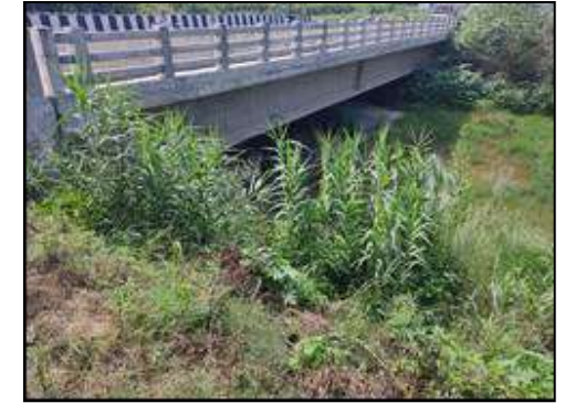
Minor Bridge at km. 66+020 (New Structure View)
