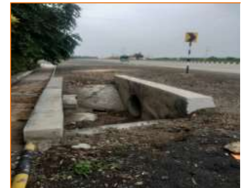
HPC at km. 70+640 (LHS)
