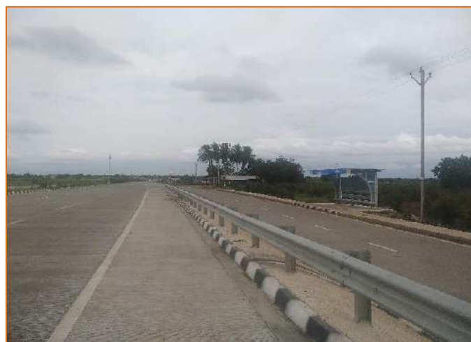
End point of Sangola Bypass at km. 299+150
