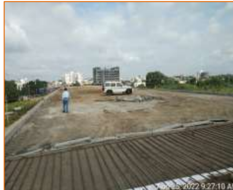
DLC & PQC of Flyover pending at km. 136.857 @ Solapur (BHS)
