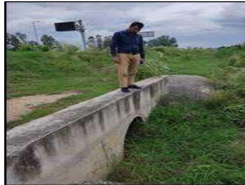
HP Culvert at km. 69+420
