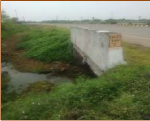
Slab culvert at km. 439+458 (LHS)
