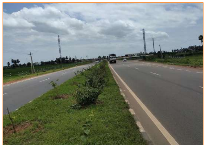
Pavement Condition at km. 57+200
