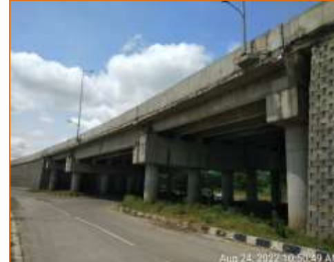
Side View of Flyover at km. 99.900 (RHS)
