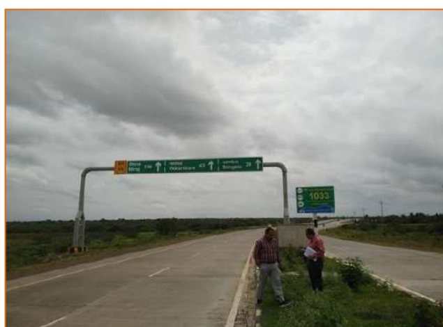
End of Project Road km. 321.600
