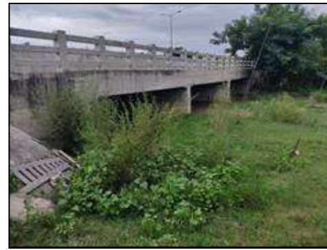
Minor Bridge at km. 72+900 (Structure View)
