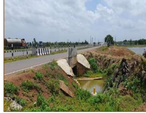
Box Culvert at km. 35+736
