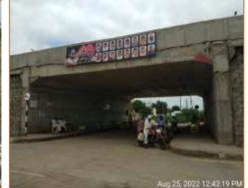
Side View of LVUP at km. 121.950 (LHS)
