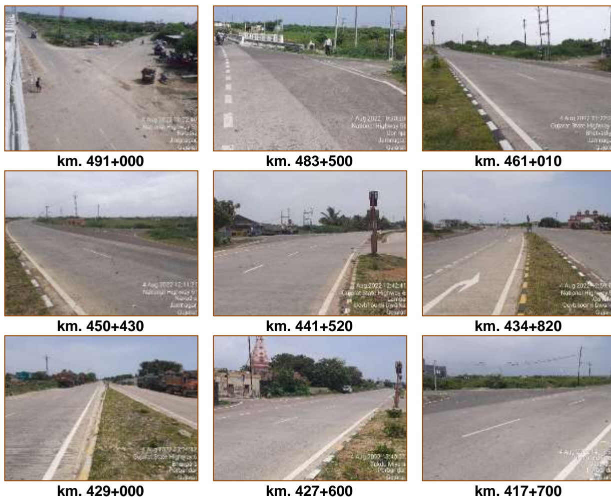
Figure 3-4 Photographs of Minor Intersection
