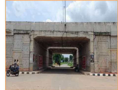
View of LVUP at km 71+140
