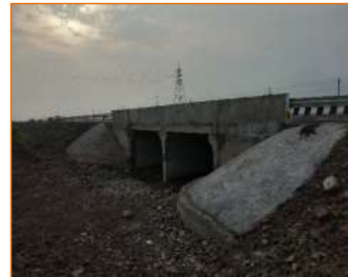
Side View of Minor Bridge at km. 47+700 (RHS)
