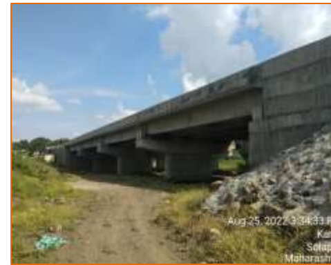
Side View of Major Bridge at km. 114.405 (RHS)
