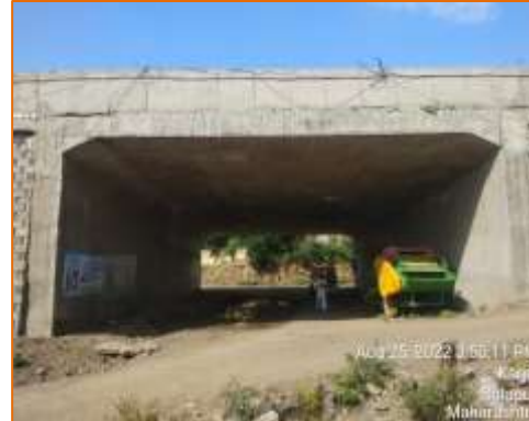
Side view of LVUP at km. 114.080 (LHS)
