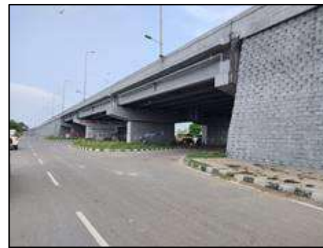
Flyover at km. 9+335
