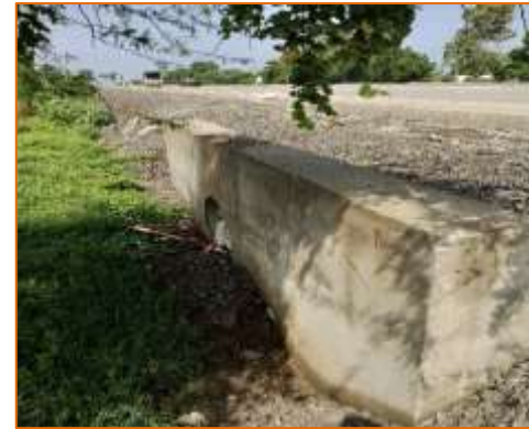
HPC at km. 32+520 (RHS)
