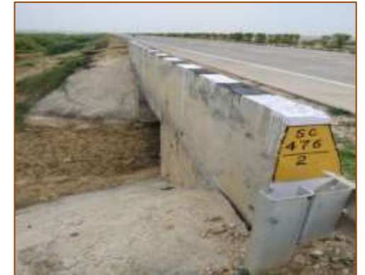
Slab culvert at km. 475+860 (RHS)
