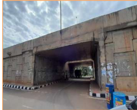
View of LVUP at km 36+420
