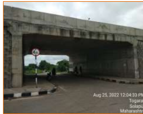
Side View of LVUP at km. 125.055 (LHS)
