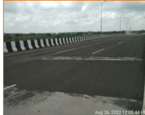
Good BC surface of Flyover at km. 103.801 (LHS)
