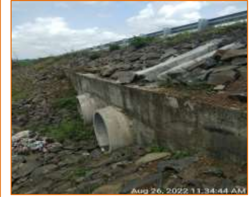
Pipe Culvert at km. 113.155-LHS (Widening)
