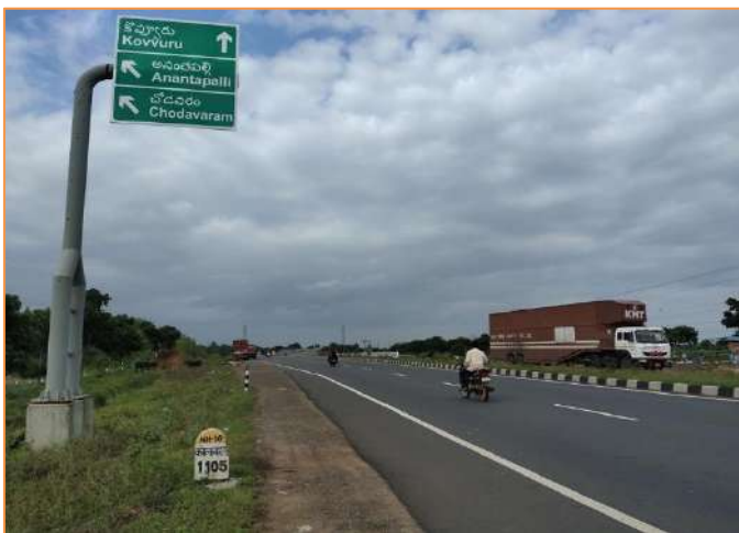
Cantilever Sign at km. 67+000
