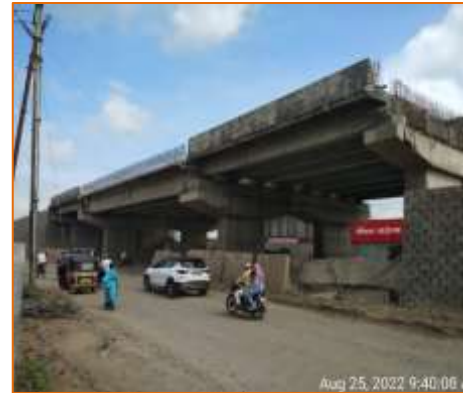
Side View of Flyover at km. 136.857 (LHS)
