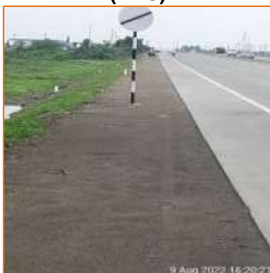
km. 53+000 to km. 54+000 (RHS)
