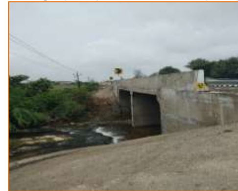
Side View of Minor Bridge at km. 54+945 (RHS)
