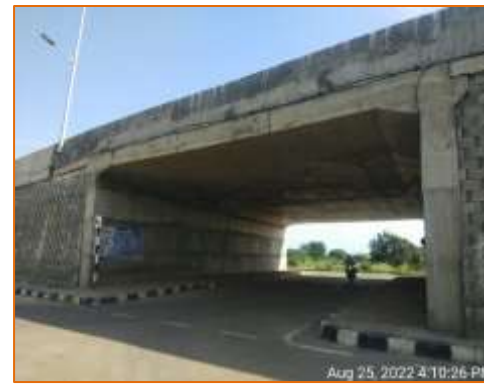
Side view of LVUP at km. 111.260 (RHS)
