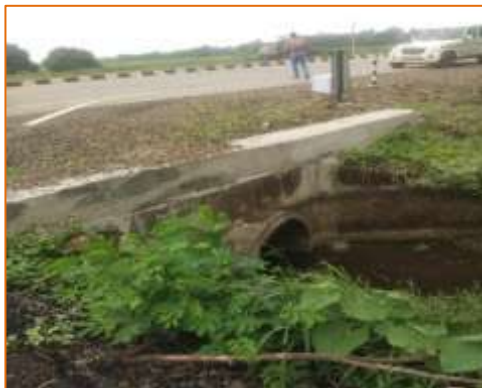
HPC at km. 66+010 (RHS)
