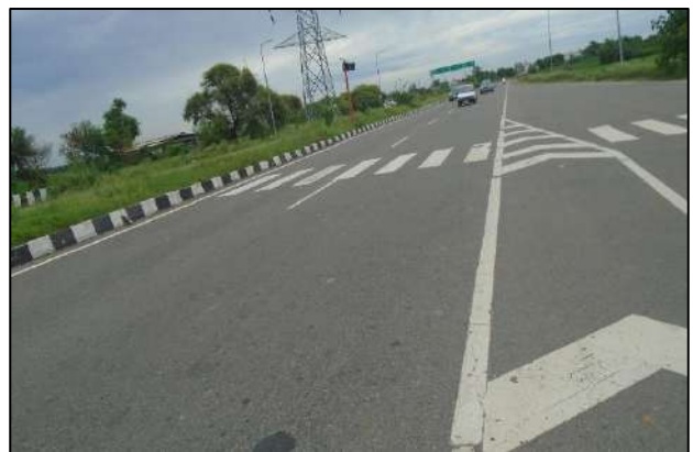
Road Marking at km. 15+800 (RHS)
