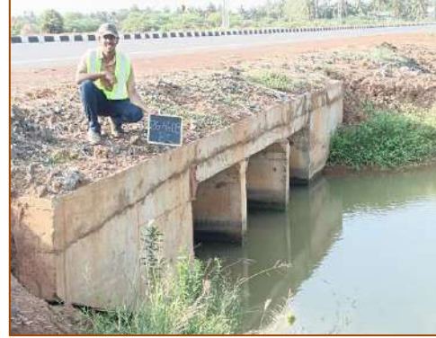
Box Culvert at km. 26+605
