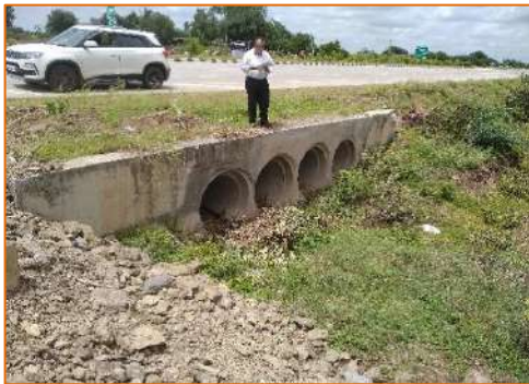
Pipe Culvert at km. 276+190
