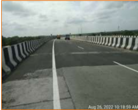
Good condition of BC surface of Flyover at km. 130.650 (RHS)
