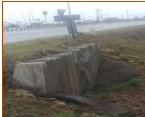
HPC at km. 437+025 (RHS)
