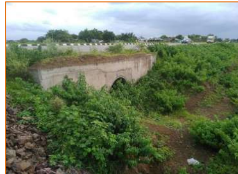
Box culvert at km. 302+500
