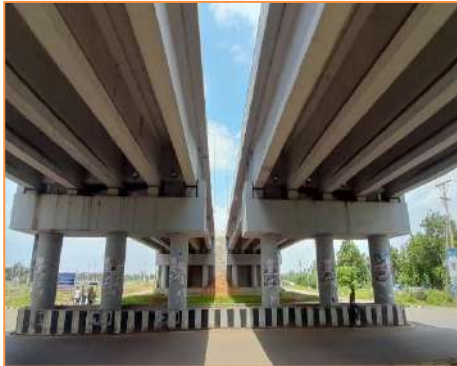
View of Flyover at km. 23+164
