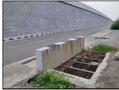
Box Culvert at km. 2+531
