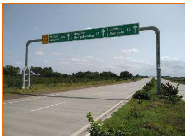
Start of Project Road at km. 276.000
