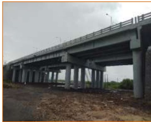
Side View of ROB at km. 0+527 (LHS)
