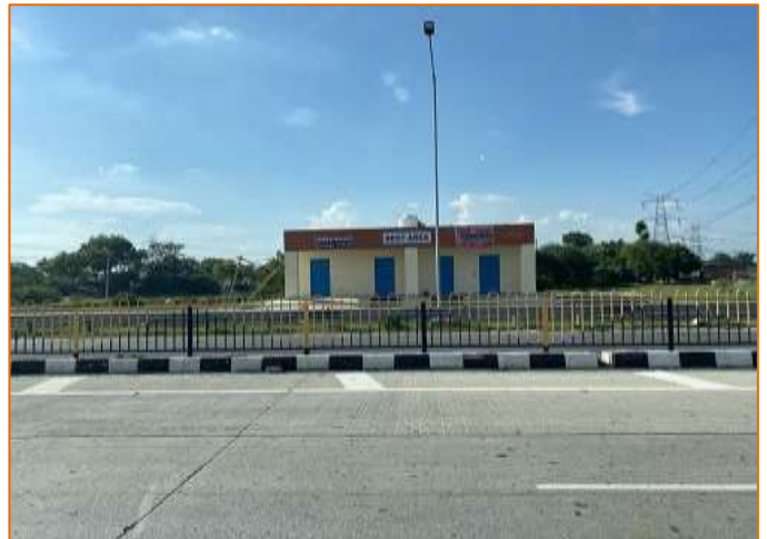
Rest Area at km. 767+500
