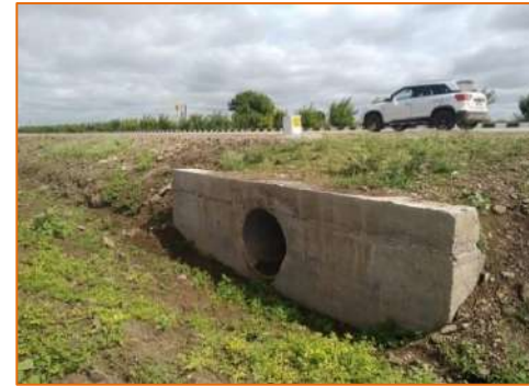
Pipe Culvert at km. 292+135
