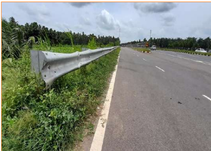
W beam Crash Barrier at km. 52+300
