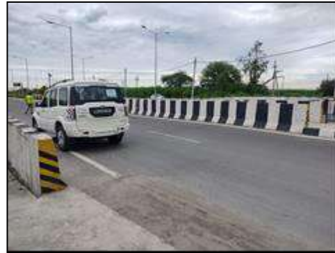
Minor Bridge at km. 77+613 (Top View)
