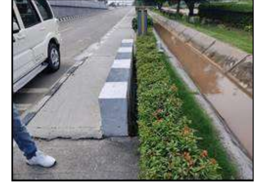
HP Culvert at km. 6+874
