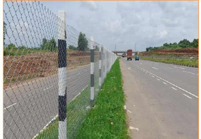
Chain fencing at km. 78+800
