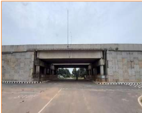
View of VUP at km 63+466
