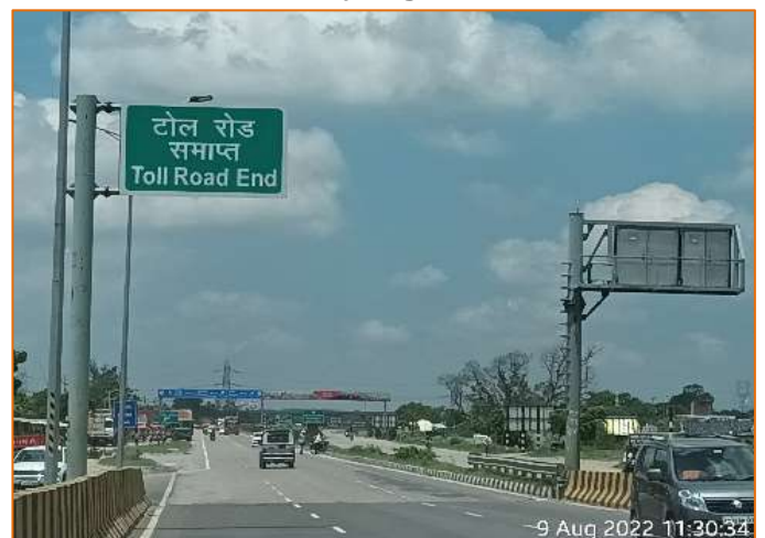
Cantilever Gantry Sign at km. 713+000.
