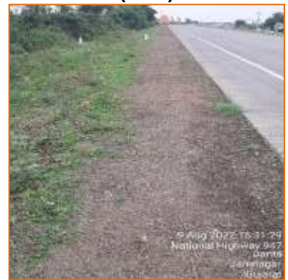
km. 64+000 to km. 63+000 (RHS)
