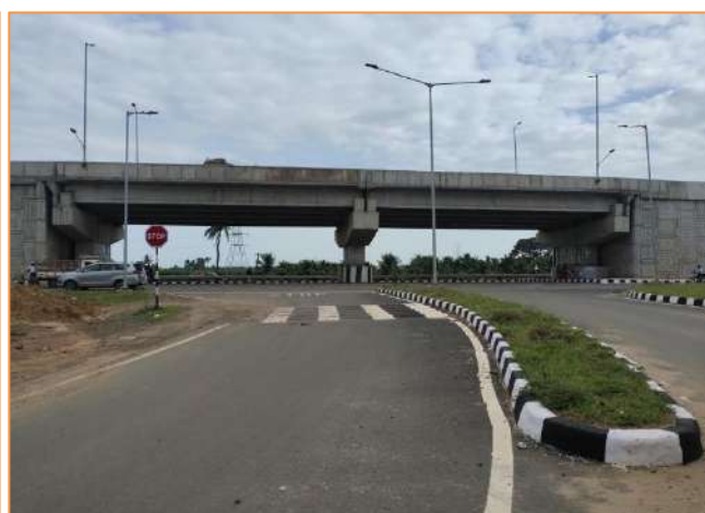
End of Project Road km. 48+830
