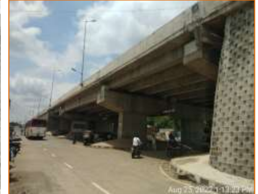
Side View of Flyover at km. 117.935 (RHS)
