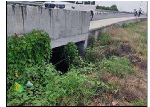
Box Culvert at km. 6+068
