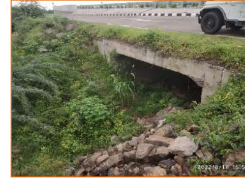
Box Culvert at km. 311.734
