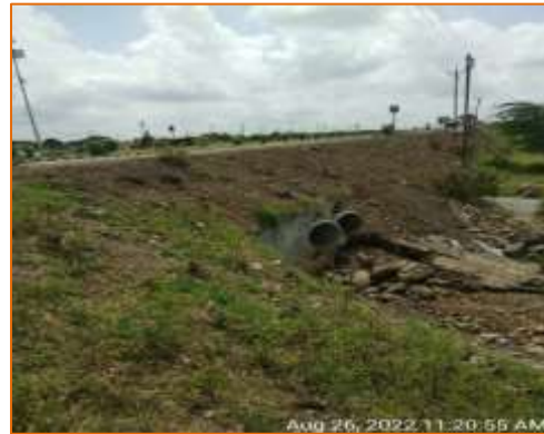
Pipe Culvert at km. 117.423 - LHS (Widening)
