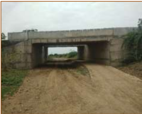
LVUP at km. 422+750 (RHS) - Under COS
