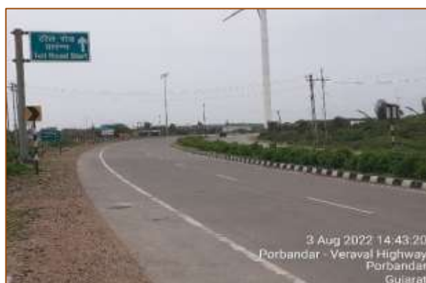
Porbandar Bypass at km. 379.100
