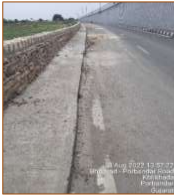
Built-up drain from km. 396+499 to km. 397+466 (LHS)
