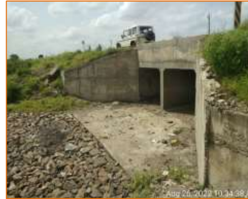
Box culvert at km. 126.643 - RHS (Reconstruction)
