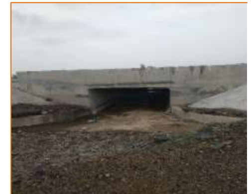
Box culvert at km. 62+720 (RHS)
