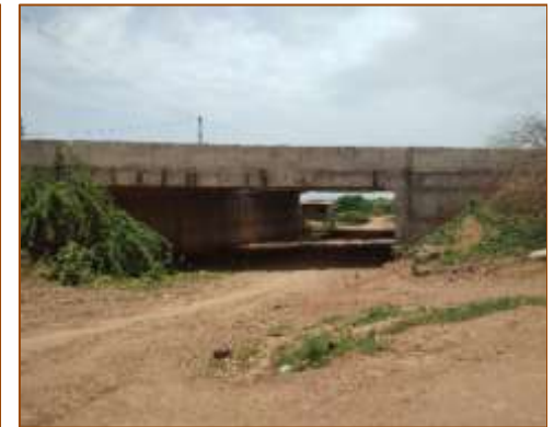
LVUP at km. 488+981 (RHS) - Under COS
