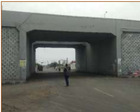
VUP at km. 400+681 (RHS)
