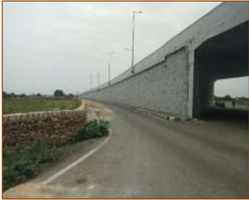
VUP at km. 397+096 (RHS) - Skew - A1 side
