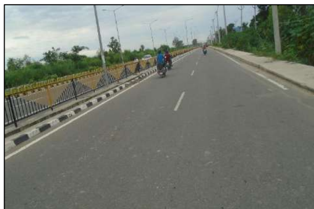
Pedestrian Guard Rail at km. 69+400
