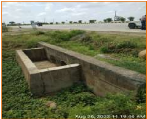
Pipe Culvert at km. 117.423 - RHS (Widening)
