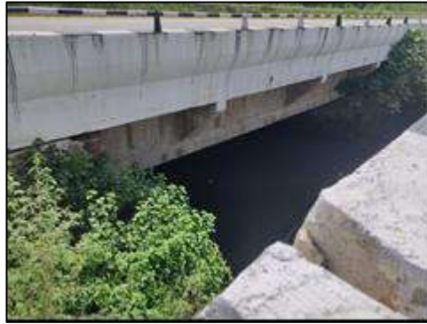
Minor Bridge at km. 62+704 (New Structure View)
