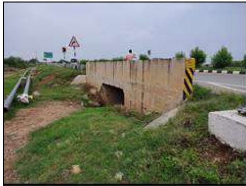
Box Culvert at km. 0+960
