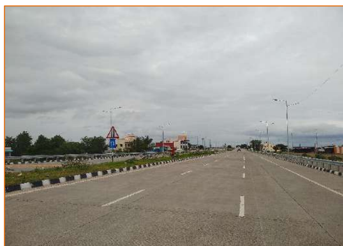
Road Markings at km. 286+600
