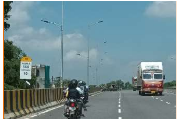
Km Stone at km. 751+000
