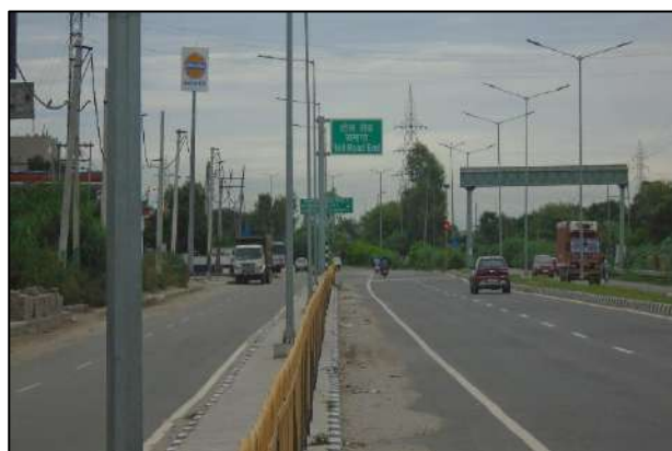
End of Project Road
