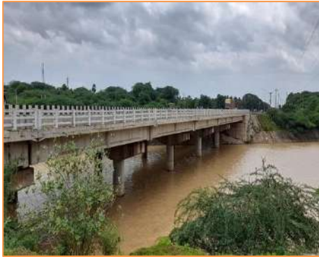
View of Major Bridge at km. 31+647
