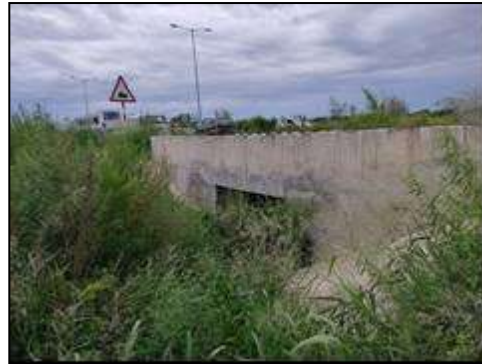
Box Culvert at km. 36+929
