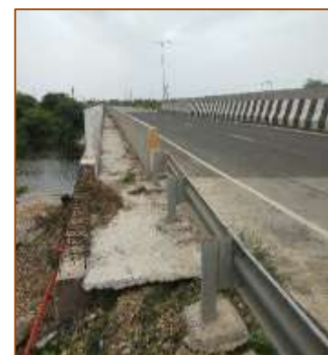
MJB at km. 456+533 (RHS)
