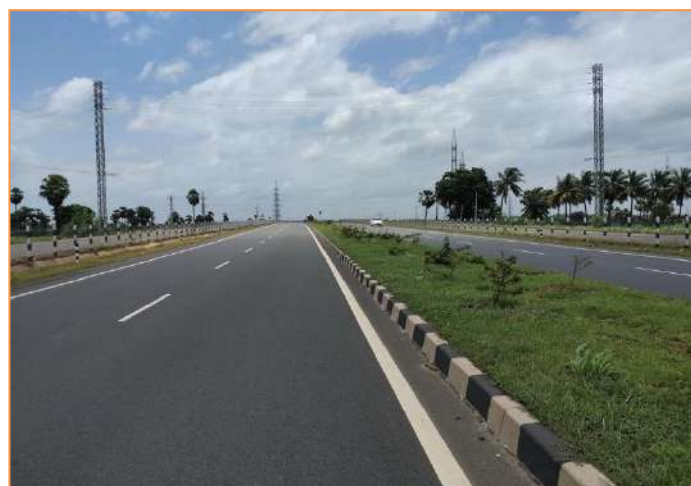
Pavement Condition at km. 76+900
