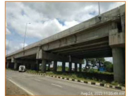
Side View of Flyover at km. 103.801 (LHS)
