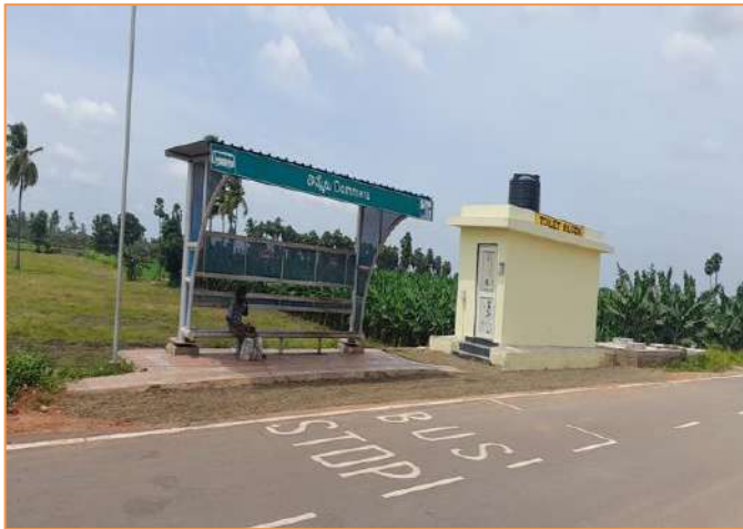
Bus Bay with Shelter at km. 79+200
