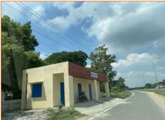
Rest Area at km. 727+800
