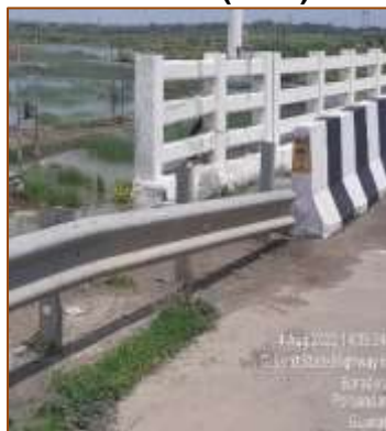
km. 416+000 to km. 417+000 (RHS)
