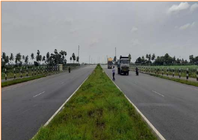
Pavement Condition at km. 41+200
