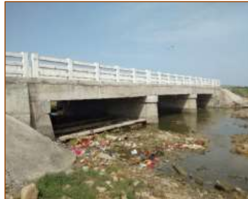
Side View of Minor Bridge at km. 494+166 (RHS) - Widening
