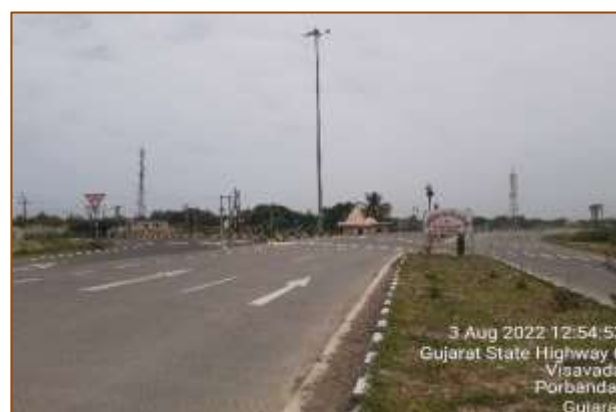
Visawada Bypass at km. 422.800
