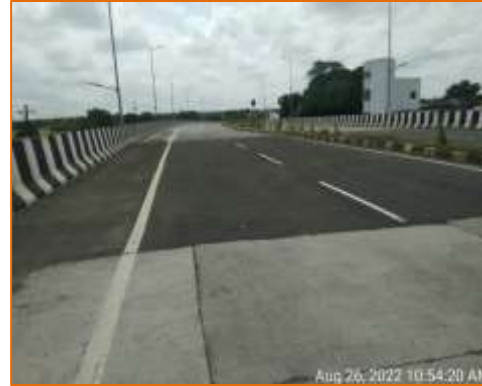
LVUP at km. 121.950 (RHS)
