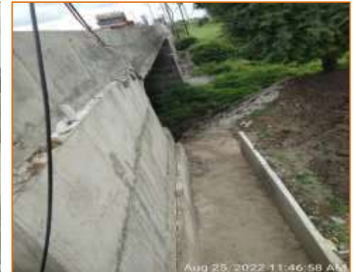
Side View of Minor Bridge at km. 130.149 - LHS (Not accessible)
