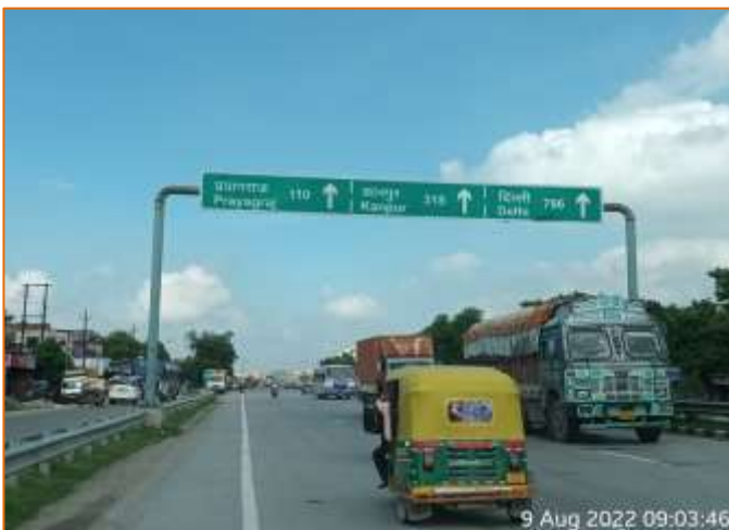
Overhead Gantry Sign at km. 785+040
