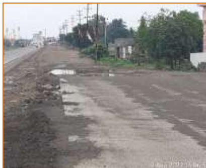
km. 56+950 to km. 56.550 (RHS)
