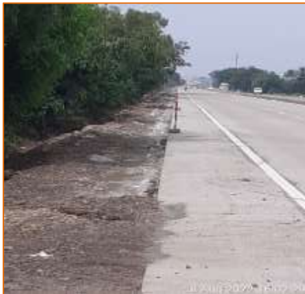
km. 32+450 Work in Progress
