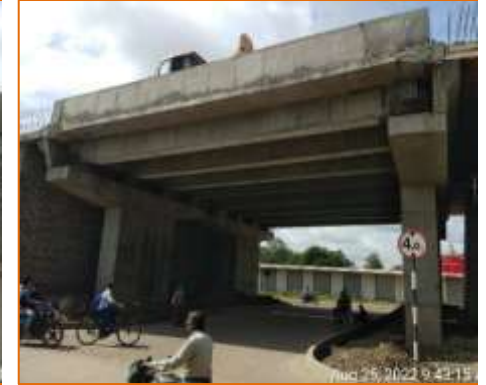
Side View of PUP at km. 136.657 (RHS)
