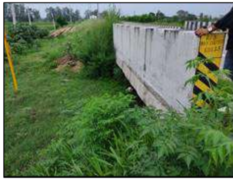
Box Culvert at km. 1+457
