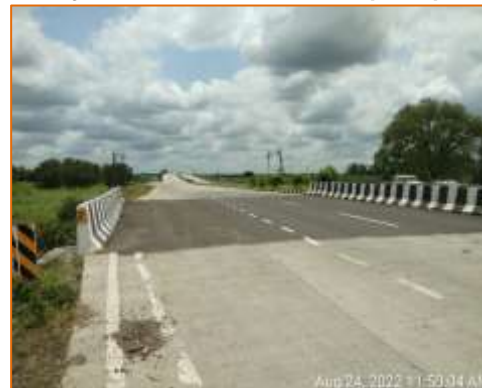
Good BC surface of Minor Bridge at km. 104.348 (RHS)
