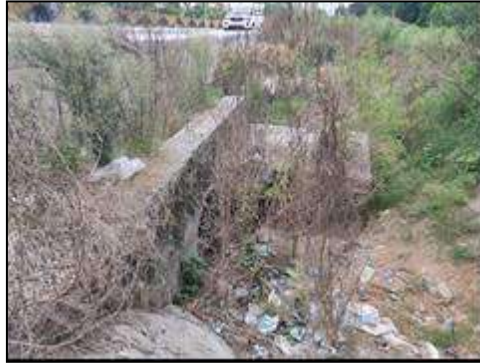
HP Culvert at km. 80+569
