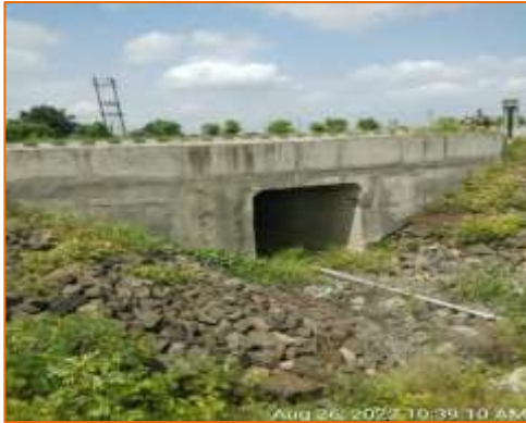
Box culvert at km. 125.495 - RHS (Reconstruction)
