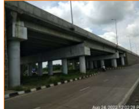
Side View of Flyover at km. 106.240 (RHS)
