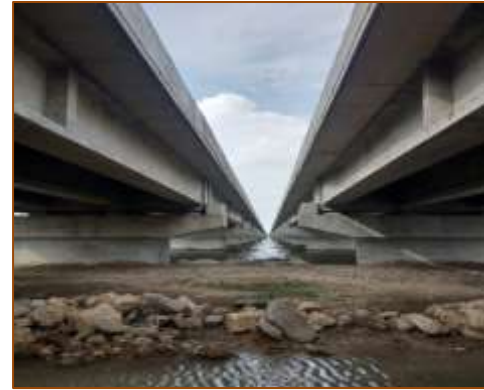
Mid Portion of MJB at km. 386+750
