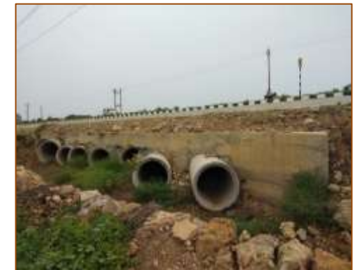
HPC at km. 456+200 (RHS)
