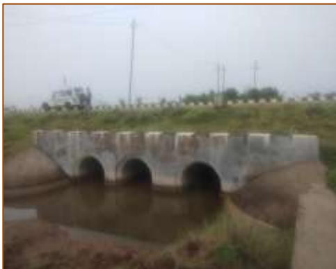
HPC at km. 437+025 (LHS)
