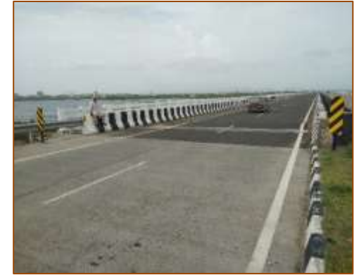
Wearing Coat of MJB at km. 386+750 (LHS)
