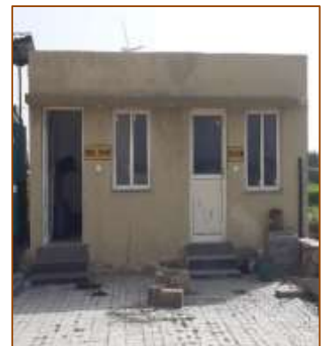
Panel / Pump Room
