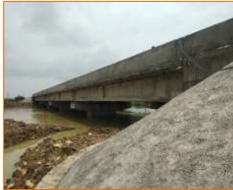
Side View of Major Bridge at km. 9+230 (LHS)
