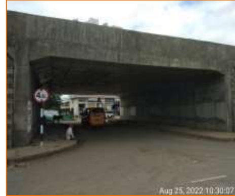
Side View of LVUP at km. 135.100 (LHS)
