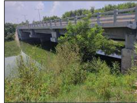
Major Bridge at km. 59+381 (New Structure View)
