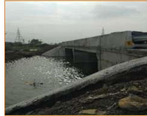
Side View of Minor Bridge at km. 40+807 (RHS)
