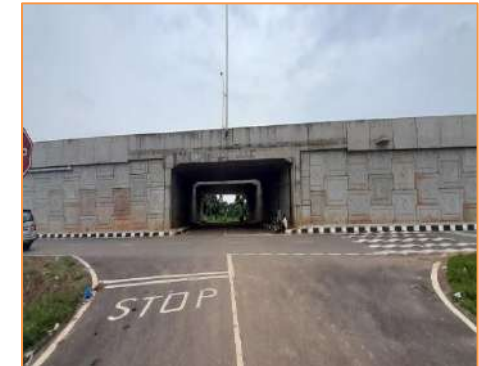
View of LVUP at km 61+932
