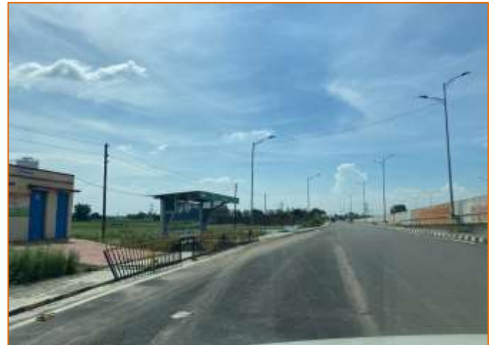
Toilet Block at km. 775+910
