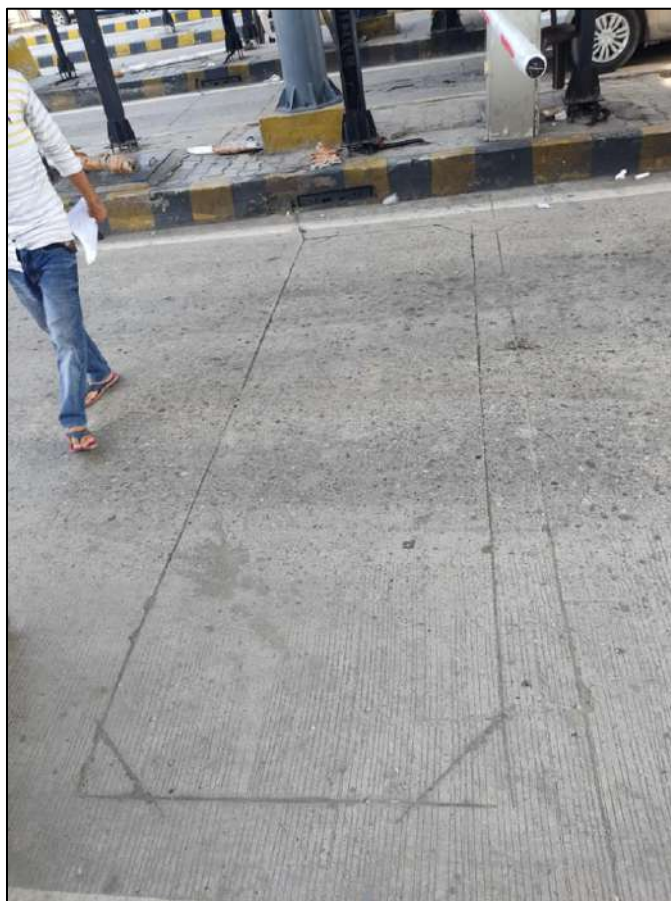
Figure 9-6 Inductive loop
