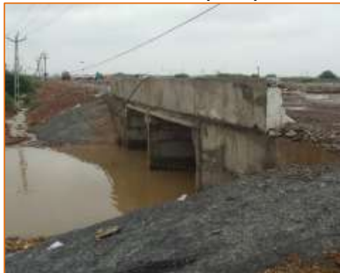
Side View of Minor Bridge at km. 13+410 (RHS)
