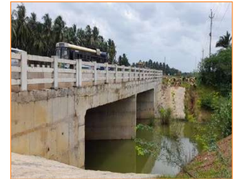
View of Minor Bridge at km. 30+774
