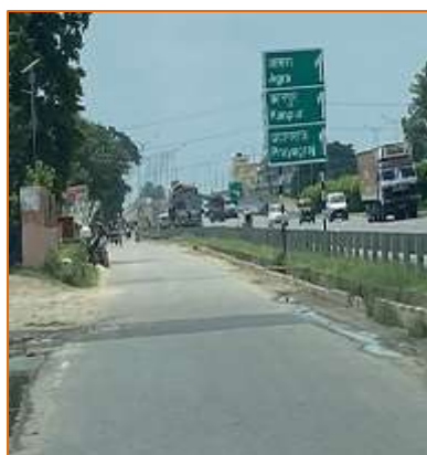
Slip Road at km. 764+700
