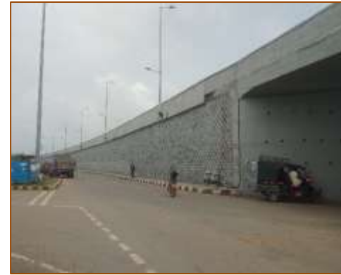
VUP at km. 432+050 (LHS) - (Miyani) under COS - RE Block Wall at A2 side
