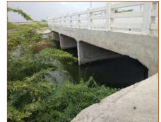
Side view of Minor Bridge at km. 406+880 (RHS) - Widening
