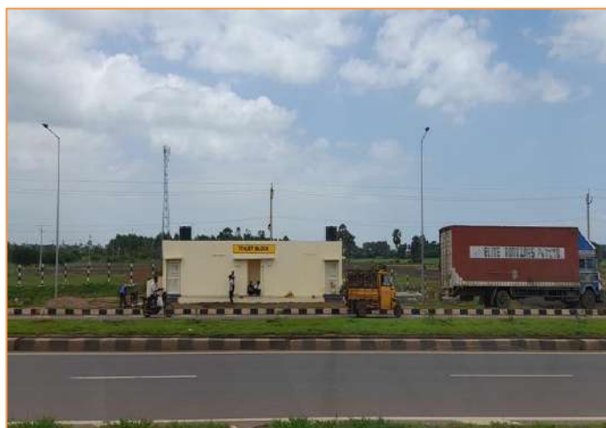
Truck Lay bye at km. 16+520
