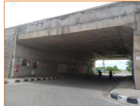
Light Vehicular Underpass at km. 285.432
