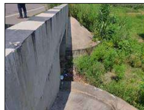
Box Culvert at km. 48+800
