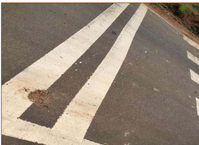
Road Markings at km. 29+400
