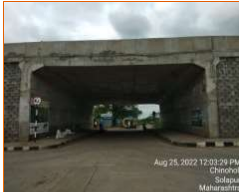
Side View of LVUP at km. 125.055 (RHS)
