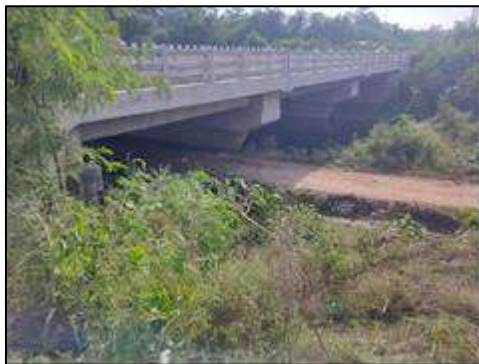
Minor Bridge at km. 71+174 (Structure View)
