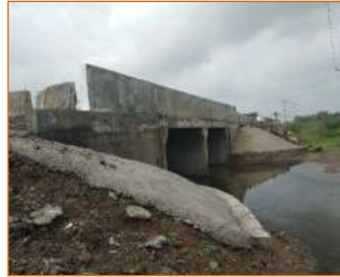
Side View of Minor Bridge at km. 51+293 (LHS)
