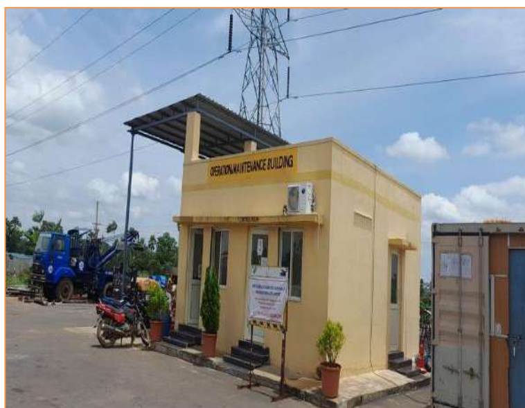
Figure 3-20 Operation and maintenance building at Toll Plaza
