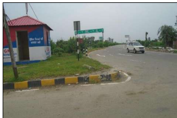
Start of Project Road - Right Carriageway
