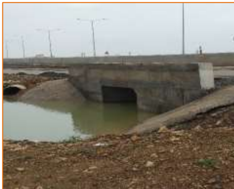
Box culvert at km. 11+950 (LHS)
