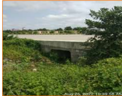
Box culvert at km. 125.495 - LHS (Reconstruction)
