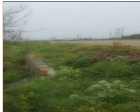
HPC at km. 437+025 (RHS)
