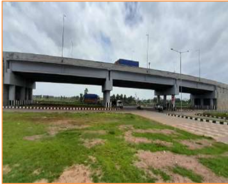
View of UDFO at km. 15+800
