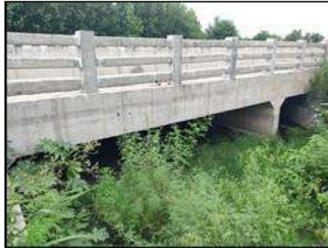
Minor Bridge at km. 74+361 (Structure View)
