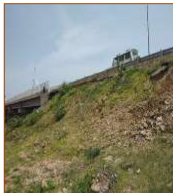
MJB at km. 415+929 (RHS)
