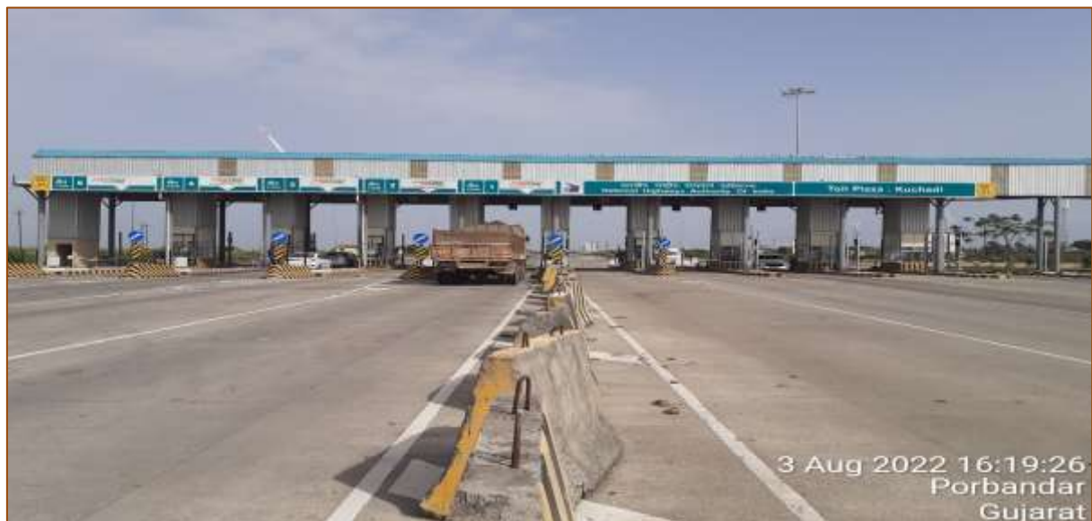
Figure 9-1 View of Kuchadi Toll Plaza (km. 409+500)
