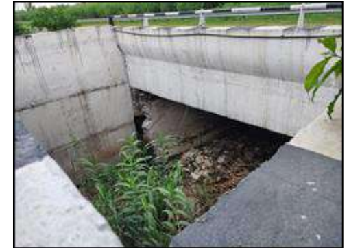
Minor Bridge at km. 76+815 (Structure View)
