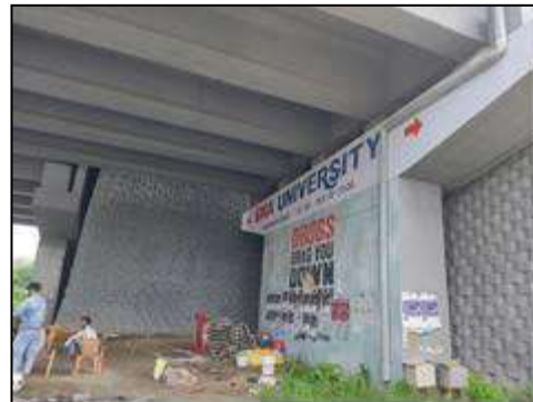
Flyover at km. 4+225
