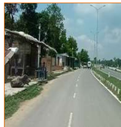
Service Road at km. 780+750
