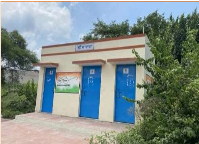
Toilet Block at km. 764+770
