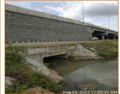
Box culvert at km. 102.650 - RHS (MCW & SR - New Construction)
