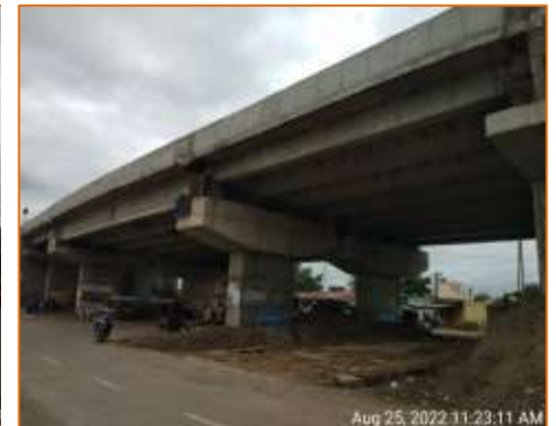
Side View of Flyover at km. 130.650 (RHS)
