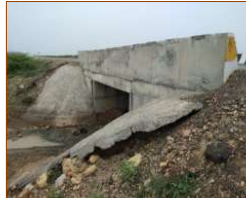
Slab culvert at km. 475+860 (LHS)
