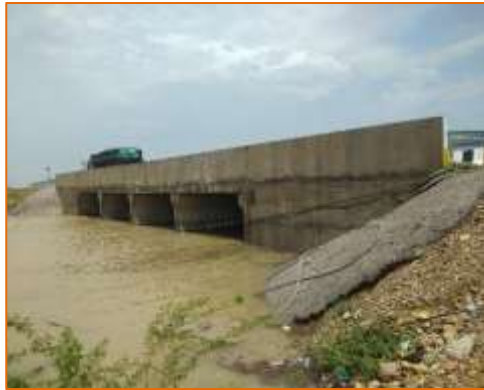
Side View of Minor Bridge at km. 3+010 (RHS)
