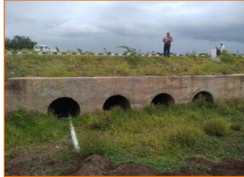
Pipe culvert at km. 317.979
