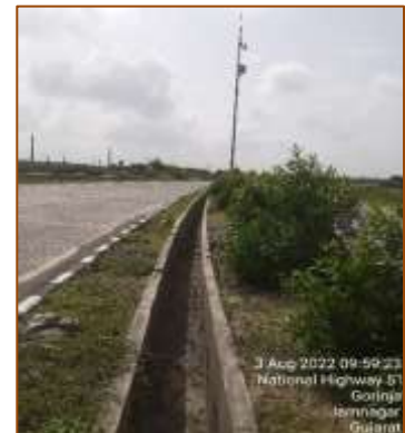
Median longitudinal drain from km. 483+000 to km. 484+000
