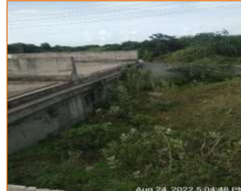
Balance work @ A1 side at km.99.586 - MNB (RHS)
