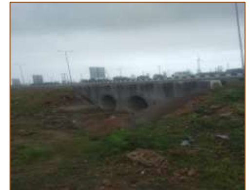
HPC at km. 409+195 (RHS)
