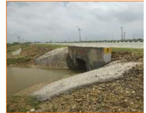
Box culvert at km. 7+240 (RHS)
