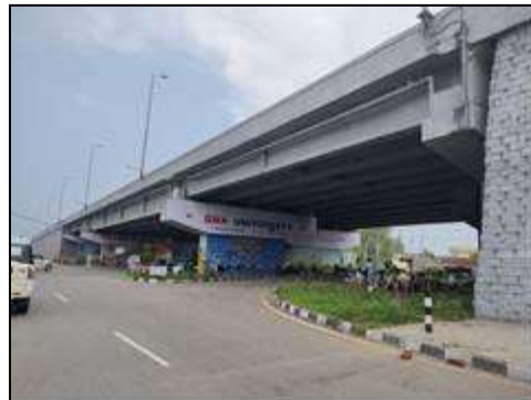
Flyover at km. 4+225
