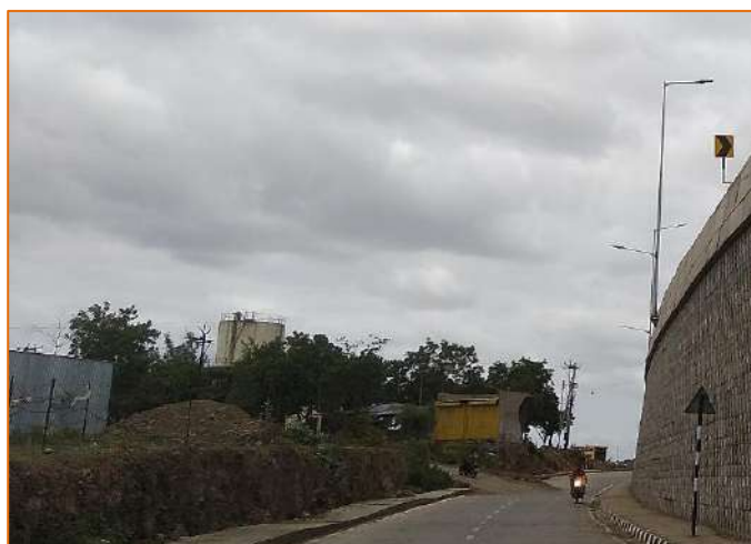
Start point of Sangola Bypass at km. 287+050
