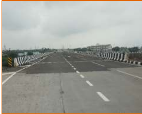
Wearing Coat of Major Bridge at km. 54+855 (LHS)
