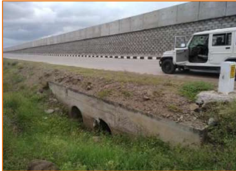
Pipe Culvert at km. 321.024
