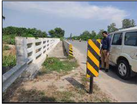
Minor Bridge at km. 66+020 (Top View)
