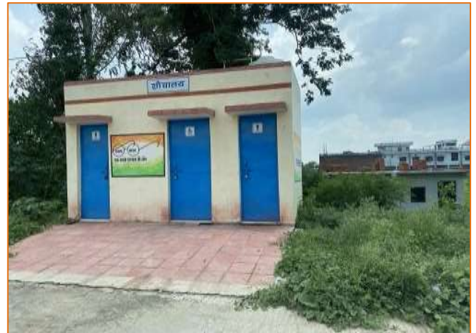
Toilet Block at km. 768+420
