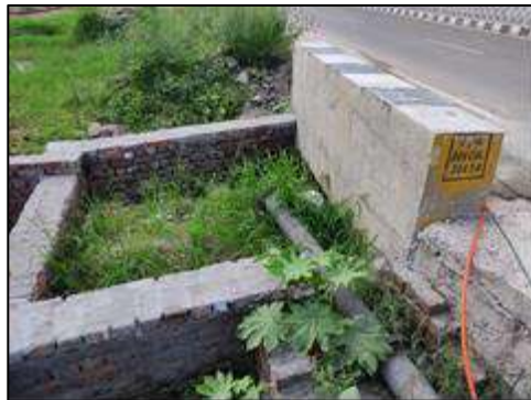
Box Culvert at km. 6+650
