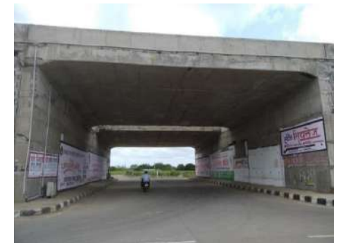
Vehicular Underpass at km. 287.300
