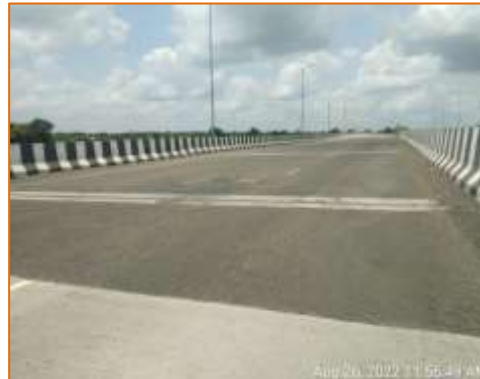
Flyover at km. 106.240 (LHS)
