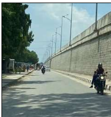
Service Road at km. 765+150
