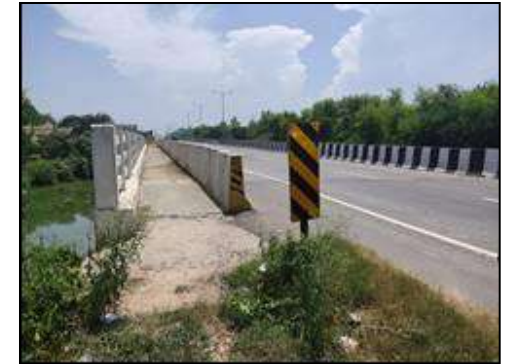
Minor Bridge at km 59+237 (top view)
