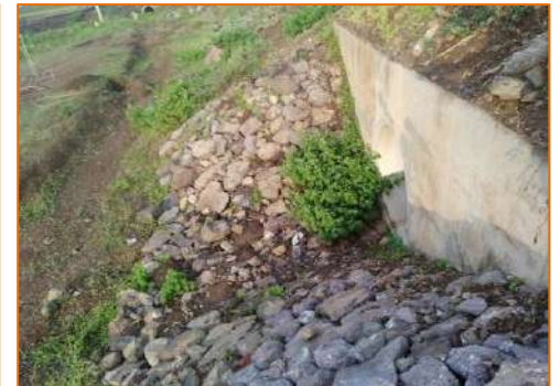
Pipe Culvert at km. 302+150
