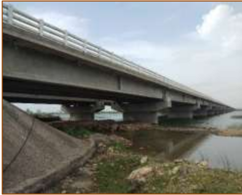
Side View of Major Bridge at km. 386+750 (RHS)
