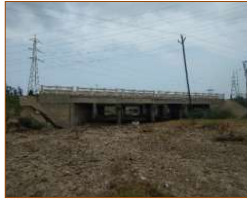
Side View of Minor Bridge at km. 462+447 (RHS) - Widening
