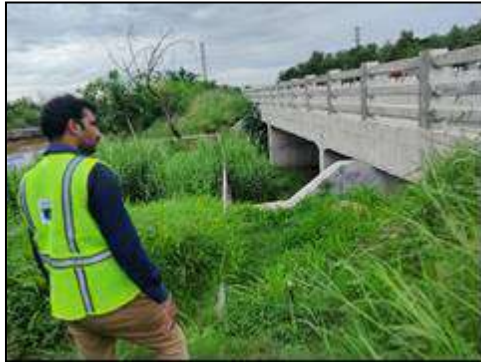
Minor Bridge at km. 74+173 (Structure View)
