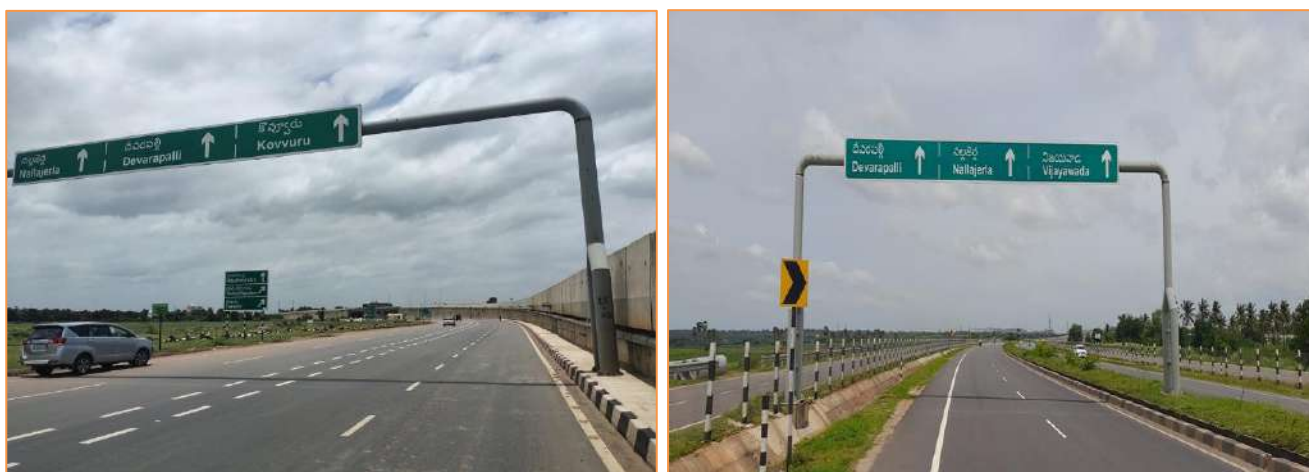
Start of Project Road at km. 15+700
