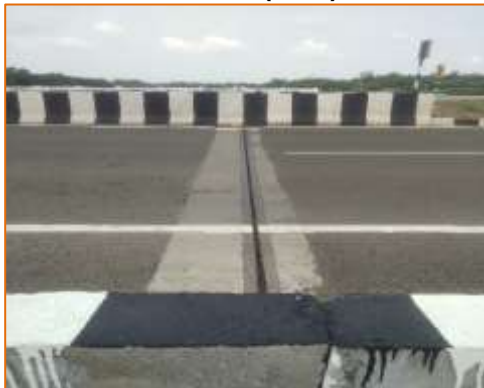
Expansion joint of Major Bridge at km. 66+310 (RHS)
