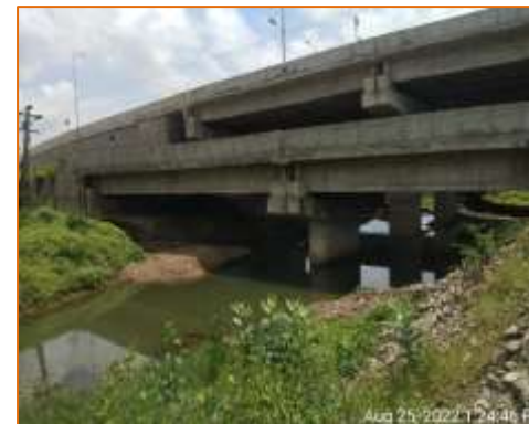
Side View of Minor Bridge at km. 117.796 - RHS (MCW & SR)
