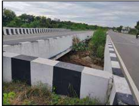
Minor Bridge at km. 72+134 (Top View)
