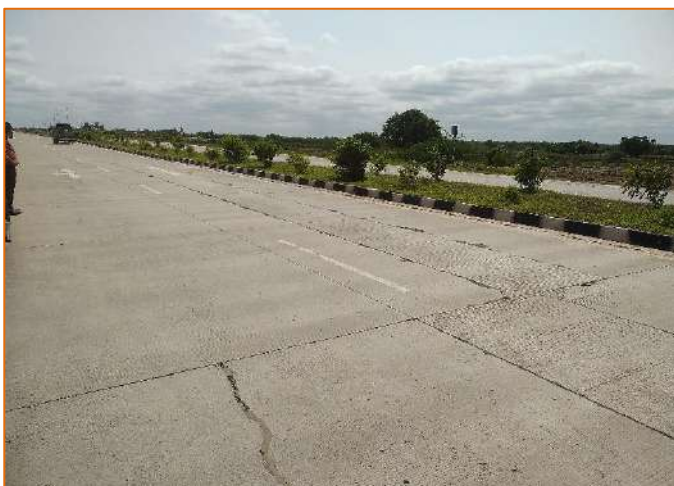
Panel Repair work done at km. 276+050 (LHS)
