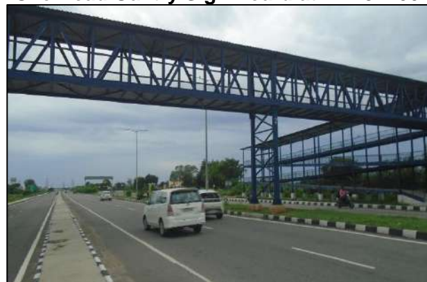
Foot Over Bridge (FOB) at km. 6+600
