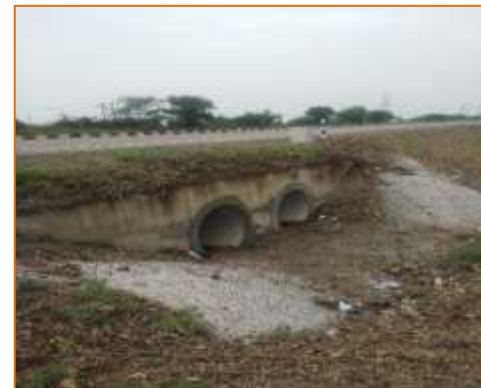
HPC at km. 70+640 (RHS)
