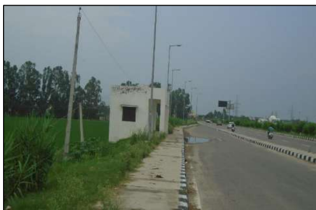
Truck Lay-Bye at km. 1+600
