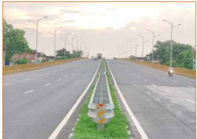
Highway Lighting at km. 740+300
