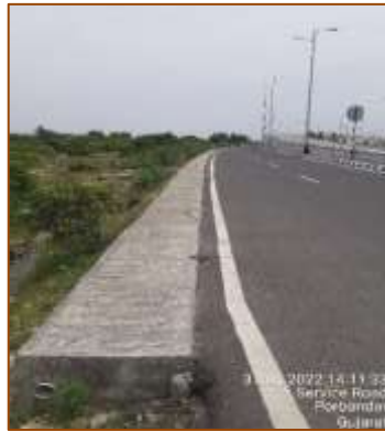
Built-up drain from km. 390+177 to km. 390+953 (RHS)
