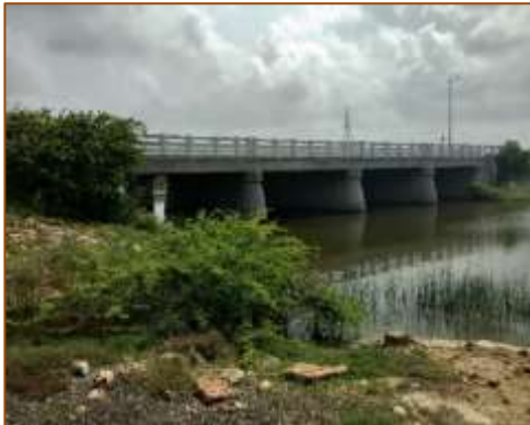
Side View of Minor Bridge at km. 492+030 (LHS) - Widening
