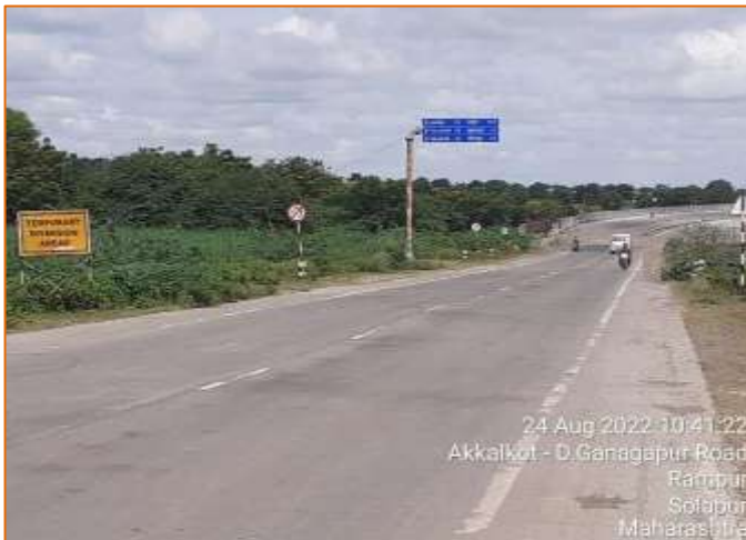
Start of the Project Highway at km. 99+400
