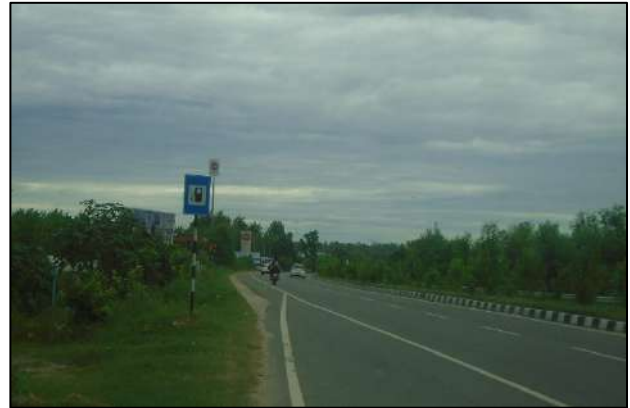
Traffic Sign Board at km. 72+000
