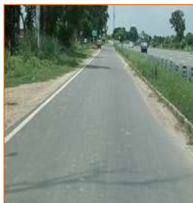
Slip Road at km. 784+400
