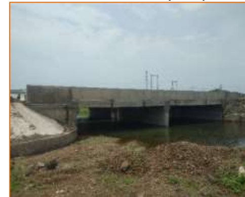
Side View of Minor Bridge at km. 67+865 (RHS)
