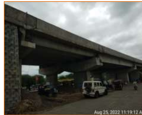
Side View of Flyover at km. 130.650 (LHS)
