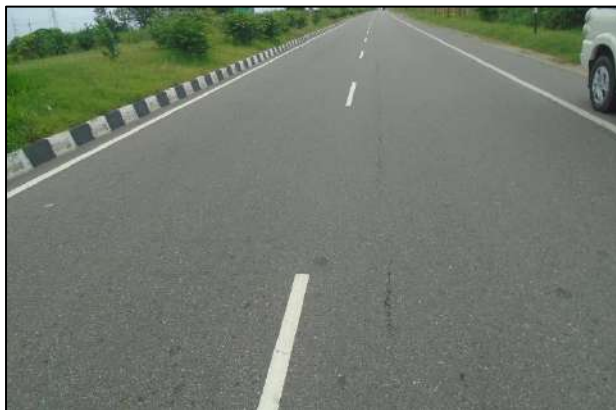
Pavement Condition at km.33+000
