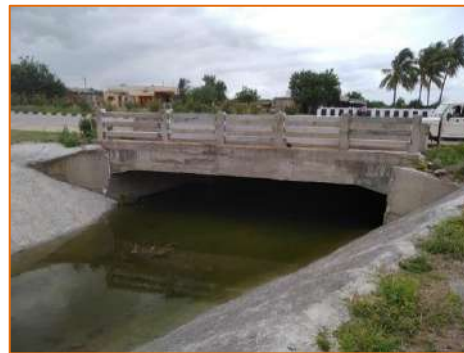
New Minor Bridge at km. 319.849 on LHS
