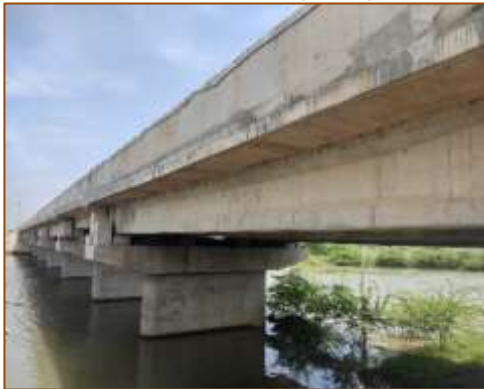
Side View of Major Bridge at km. 420+180 (LHS)
