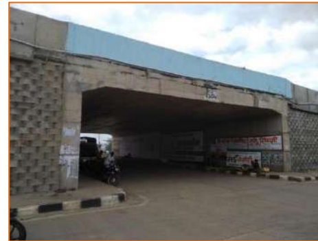
Light Vehicular Underpass at km. 283.165
