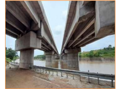
View of Major Bridge at km. 68+742
