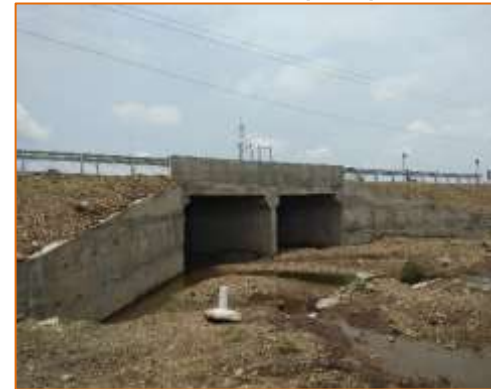
Side View of Minor Bridge at km. 64+765 (RHS)
