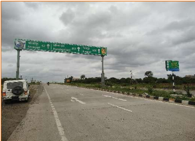
Cantilever Gantry Sign at km. 321+600
