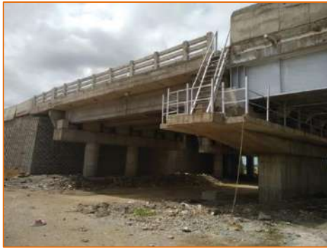
Rail Over Bridge at km. 294.125
