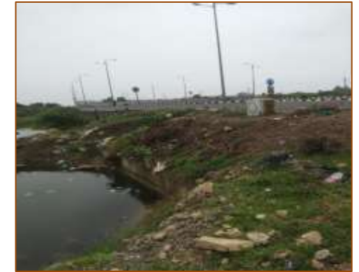
HPC at km. 391+096 (RHS)
