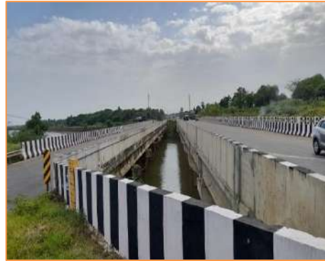
View of Major Bridge at km. 48+222
