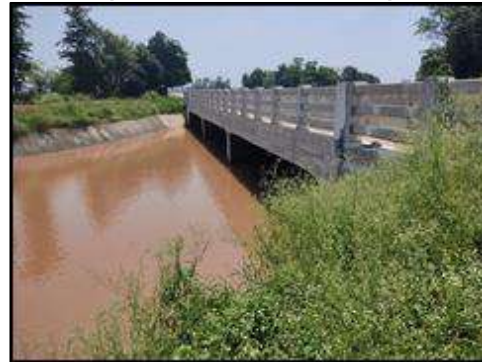
Minor Bridge at km. 48+323 (New Structure View)
