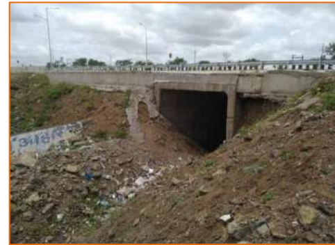
Box Culvert at km. 284+112
