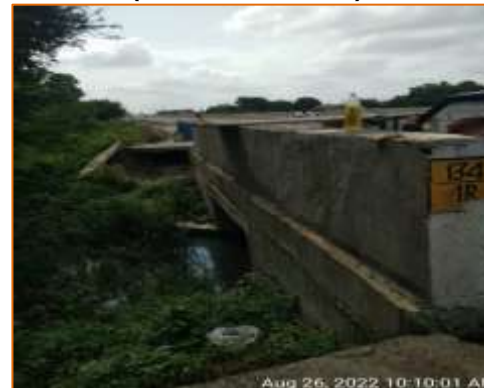
Box culvert at km. 133.524 - RHS (Reconstruction)
