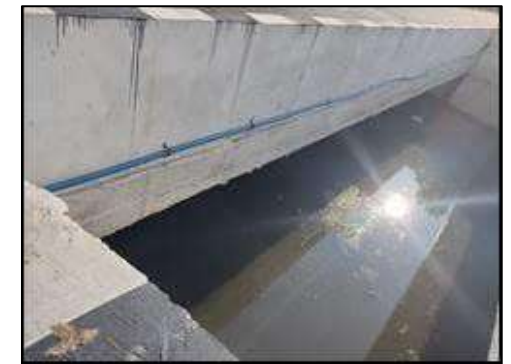
Minor Bridge at km. 71+727 (Structure View)
