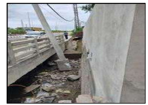
Minor Bridge at km. 80+045 (Structure View)
