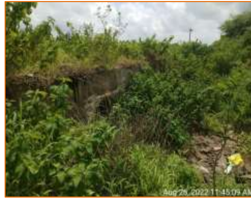
Pipe Culvert at km. 109.578 - LHS (Widening)
