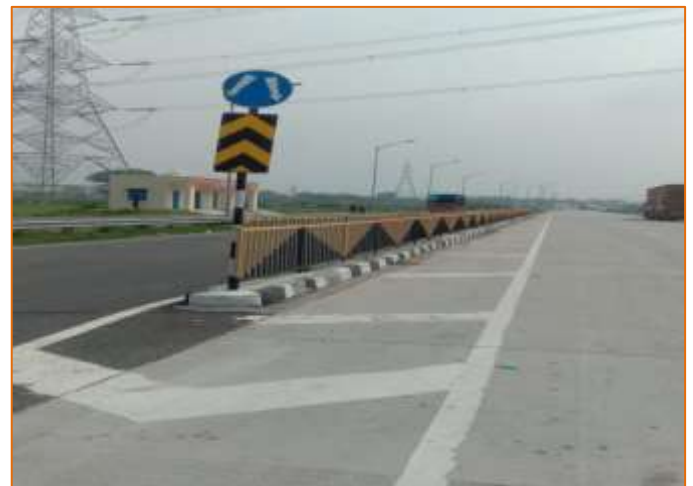
Pedestrian Guard Rail at km.766+600
