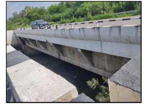
Minor Bridge at km. 63+615 (New Structure View)
