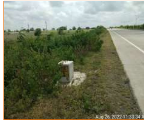
Pipe Culvert at km. 113.155 - RHS (Widening)
