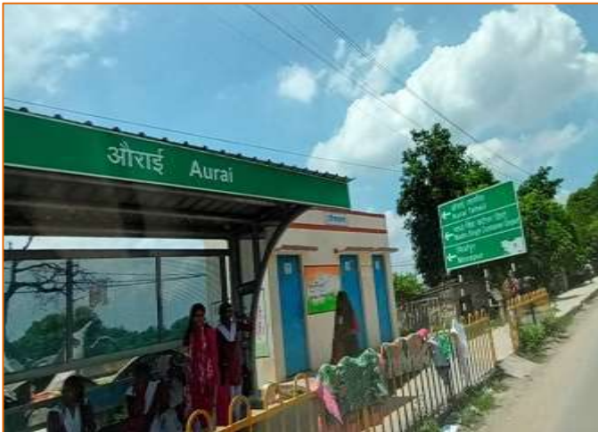
Toilet Block at km. 754+130
