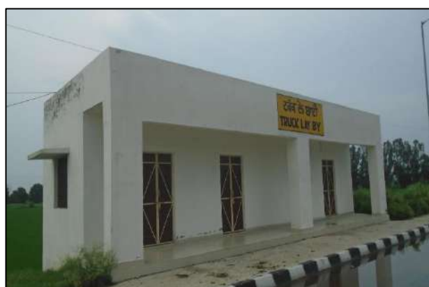
Truck Lay-Bye at km. 1+600
