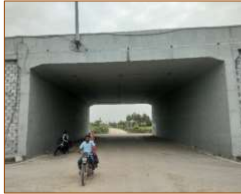
LVUP at km. 381+600 (LHS) - Under COS
