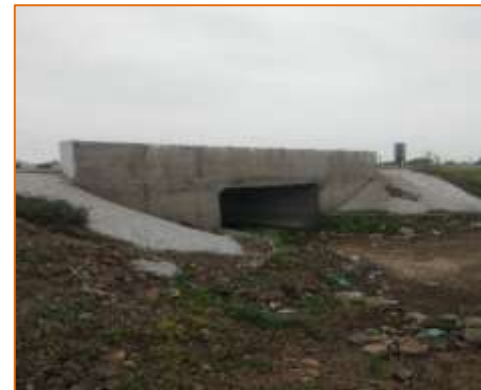
Box culvert at km. 62+720 (LHS)
