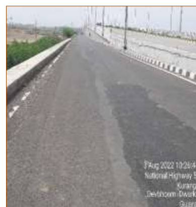
km. 467+601 to km. 468+347 (RHS)
