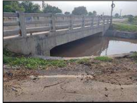
Minor Bridge at km. 35+812 (New Structure View)
