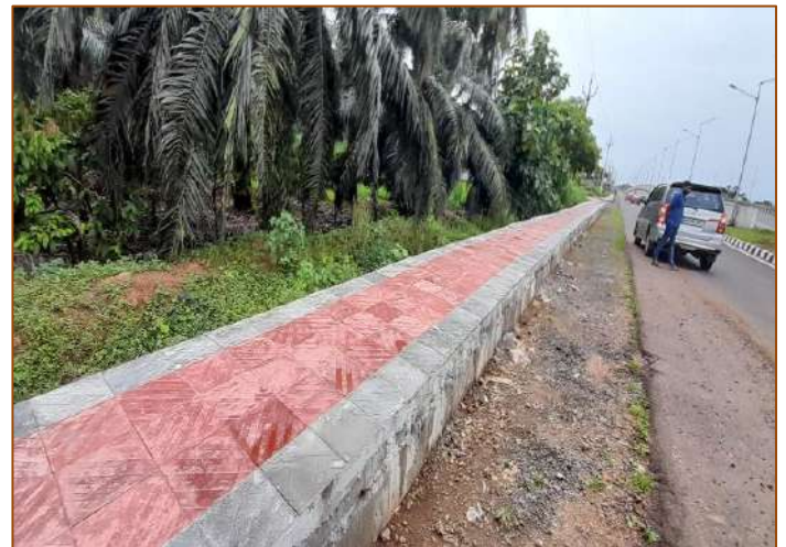
Built-up Drain cum footpath at km. 36+450
