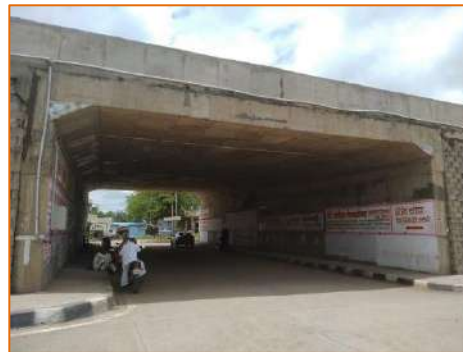
Light Vehicular Underpass at km. 278.700
