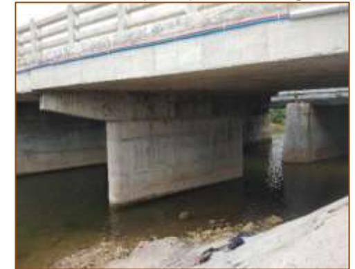
Bottom of Minor Bridge at km. 455+195 (RHS)
