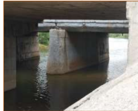
Bottom of Minor Bridge at km. 455+195 (BHS)
