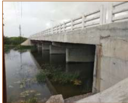
Side View of Minor Bridge at km. 459+038 (RHS) - Widening
