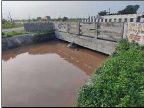
Minor Bridge at km. 35+812 (Existing Structure View)
