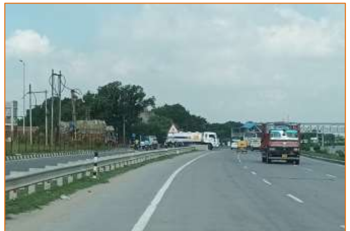
Crash Barrier at km. 782+000
