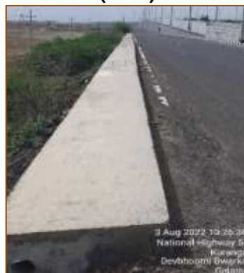
Built-up drain from km. 467+601 to km. 468+347 (RHS)
