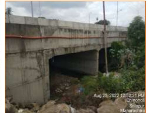
Side View of Minor Bridge at km. 121.678 (RHS)
