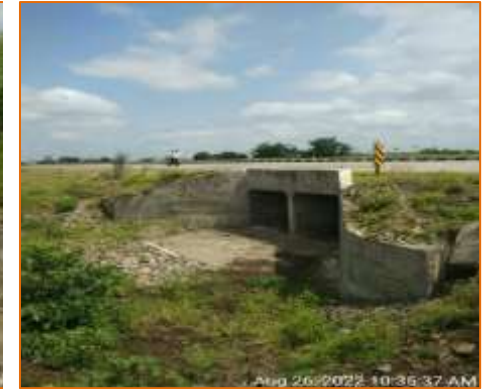
Box culvert at km. 126.643 - LHS (Reconstruction)
