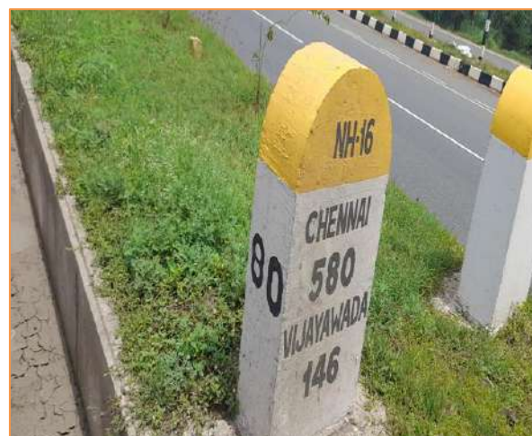
kilometer stone at km 80+000
