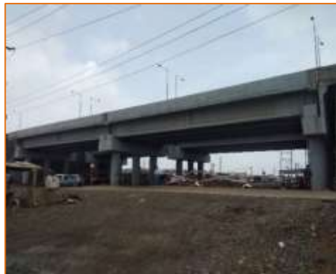
Side View of VUP at km. 12+420 (LHS)
