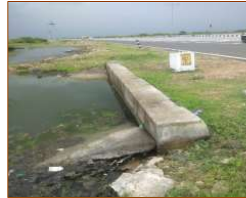
HPC at km. 391+096 (LHS)
