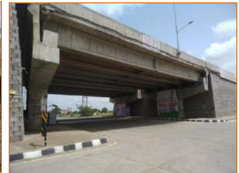
Vehicular Underpass at km. 290.700
