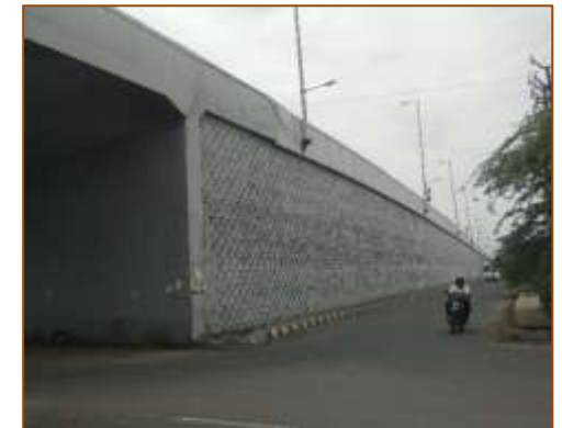
VUP at km. 400+681 (LHS) at A1 side
