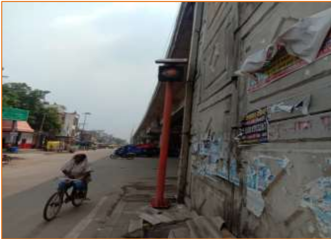
LED Blinker at km. 741+010
