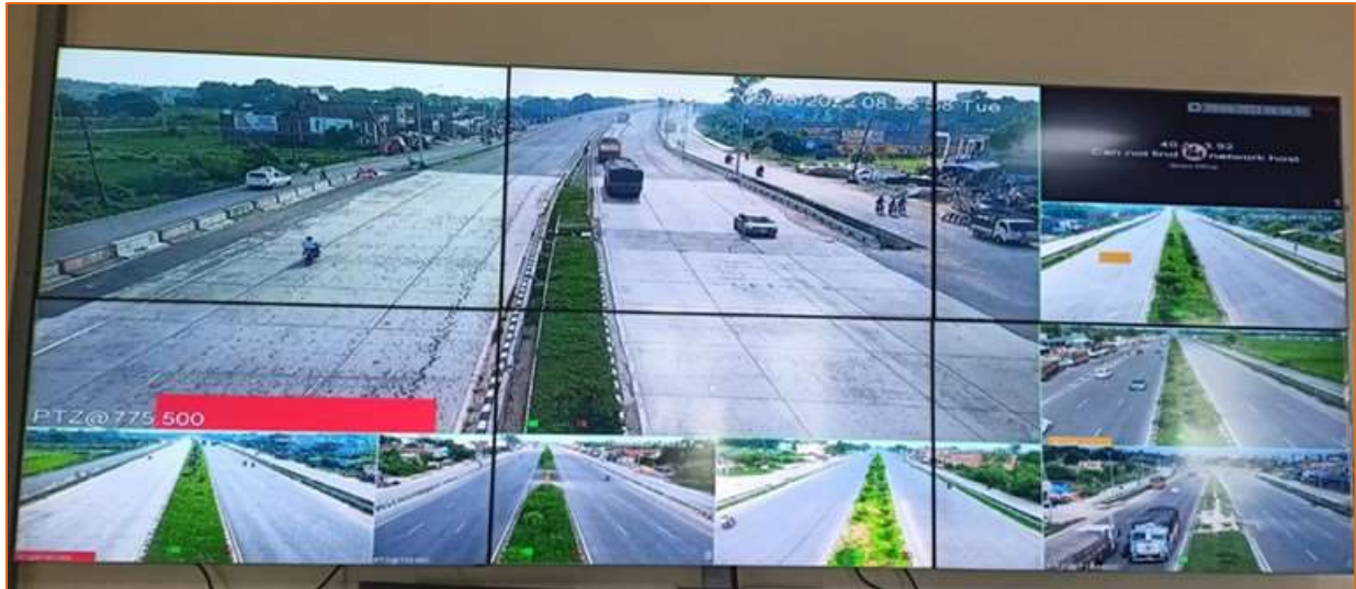
Figure 9-10 Video wall in ATMS control centre
