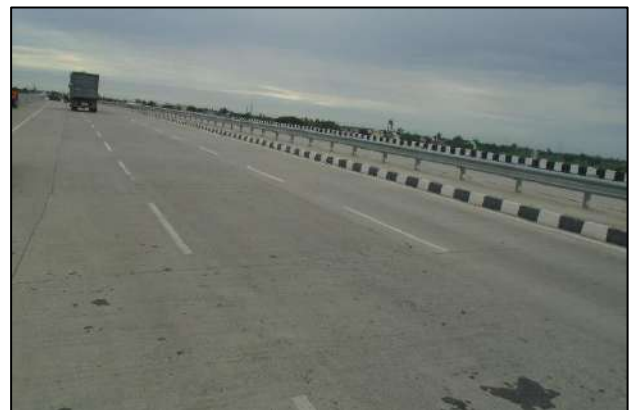
Crash Barrier at curve location
