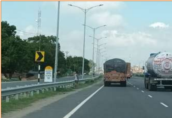
Km Stone at km. 776+000
