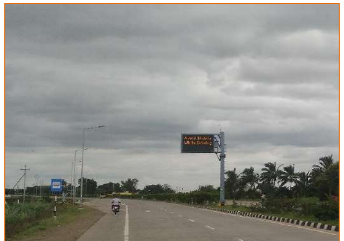
VMS Board at km. 301+100
