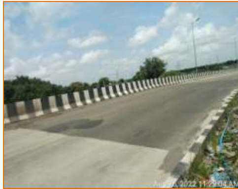
LVUP at km. 114.080 (LHS)
