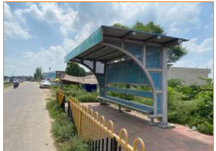
Bus Shelter at km. 767+915
