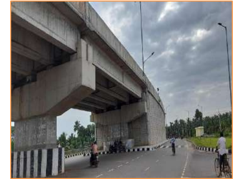
View of UDFO at km. 48+830
