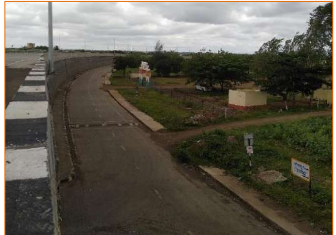
Built-up Drain at km. 299+350
