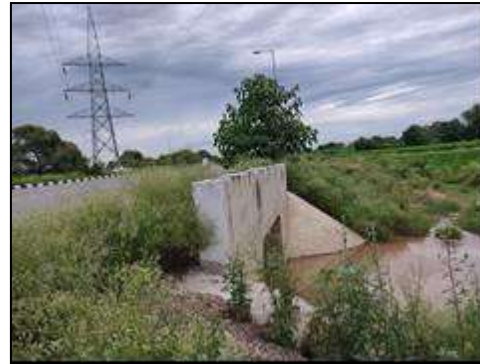
Box Culvert at km. 17+946
