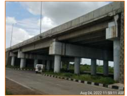
Side View of Flyover at km. 106.240 (LHS)
