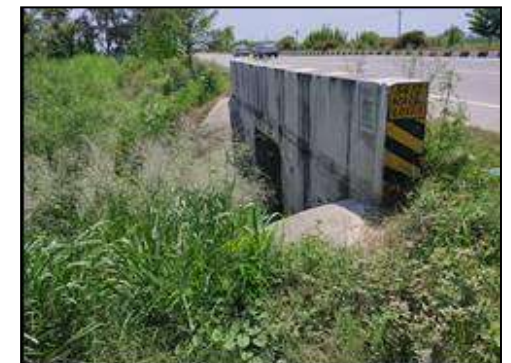
Box Culvert at km. 53+510
