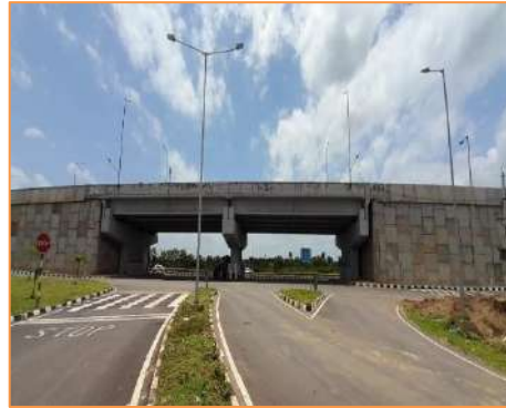
View of UDFO at km. 20+440
