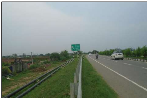
Crash Barrier at high embankment
