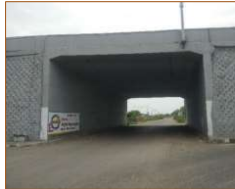
VUP at km. 396+865 (RHS)
