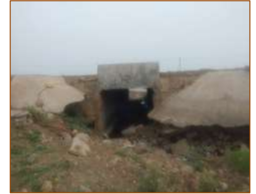
Slab culvert at km. 441+648 (RHS)
