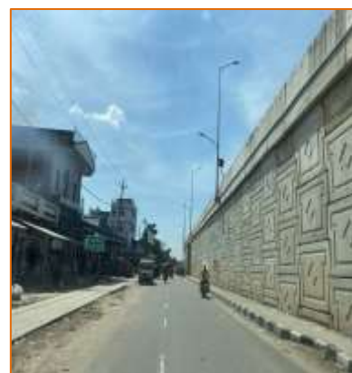
Service Road at km. 734+175
