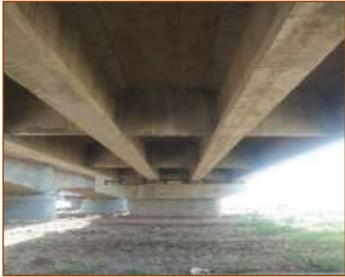
Bottom of MJB - New at km. 433+276 (LHS)
