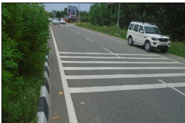
Road Marking at km. 70+000 (RHS)
