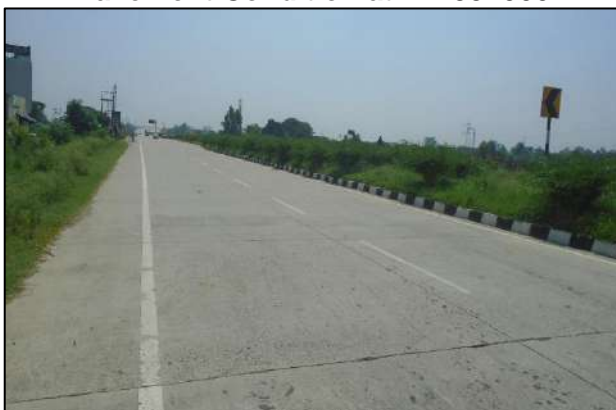
Rigid Pavement at km. 38+000
