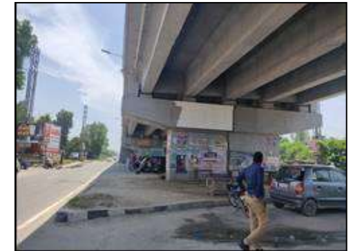
Flyover at km. 59+818
