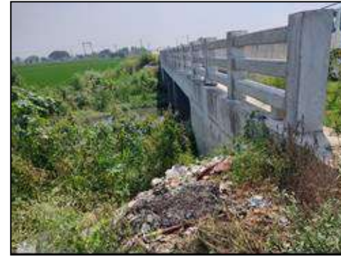
Minor Bridge at km. 38+326 (New Structure 4-lane View)
