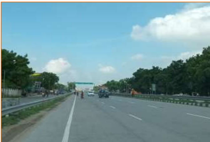
Crash Barrier at km. 785+240
