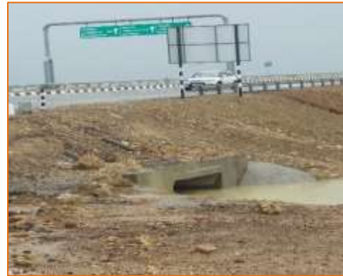
Box culvert at km. 0+060 (RHS)
