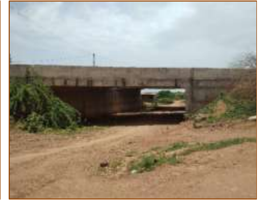
LVUP at km. 488+981 (RHS) - Under COS
