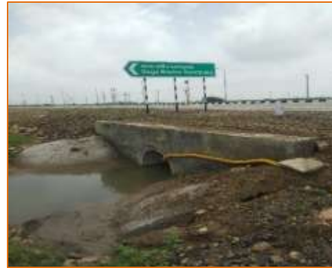
HPC at km. 5+800 (LHS)
