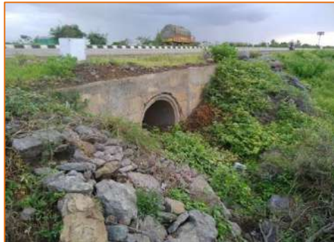
Pipe culvert at km. 304+300
