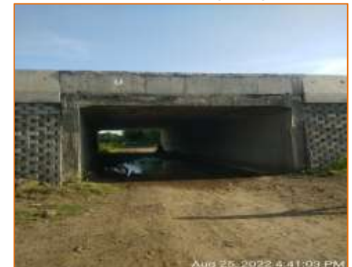
Side View of PUP at km. 104.820 (RHS) - Under COS
