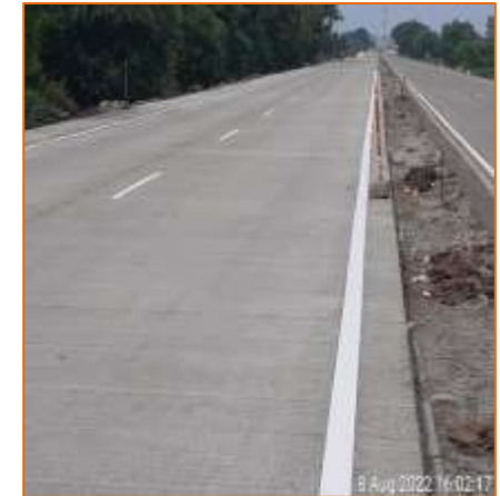
km. 32+450 Work in Progress
