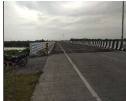
Top View of MJB - Widening at km. 420+180 (LHS)
