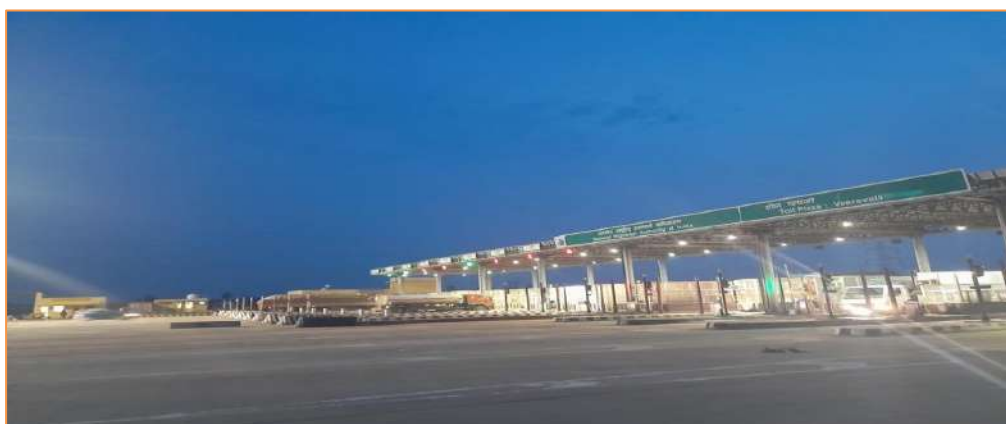
Figure 3-13 View of Toll Plaza
