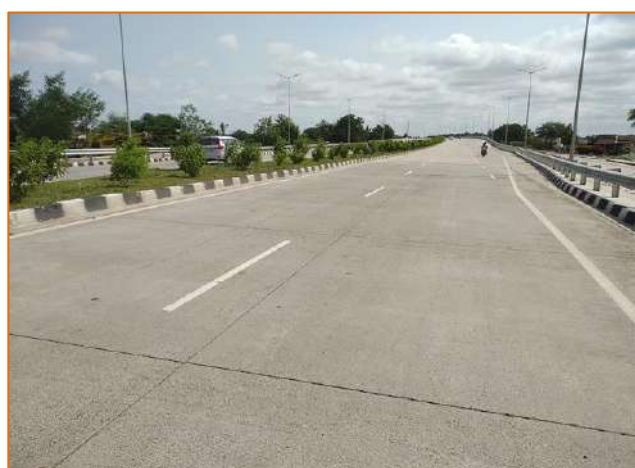
Start of Project Road at km. 276.000
