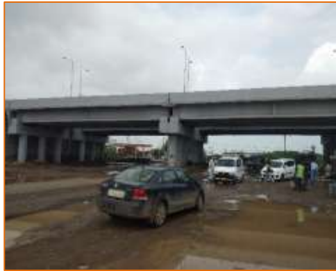
Side View of VUP at km. 12+420 (RHS)
