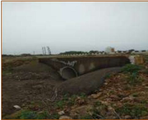
HPC at km. 380+328 (LHS)
