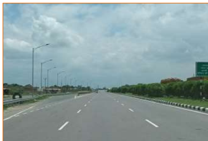
Truck Lay Bye at km. 767+330
