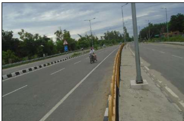
Pedestrian Guard Rail at km. 69+400
