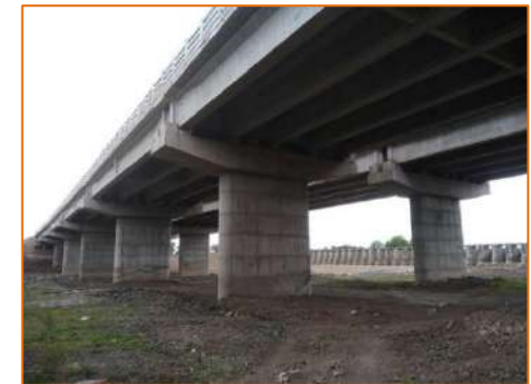
New Major Bridge Bottom View of Girder and Pier at km. 280.420
