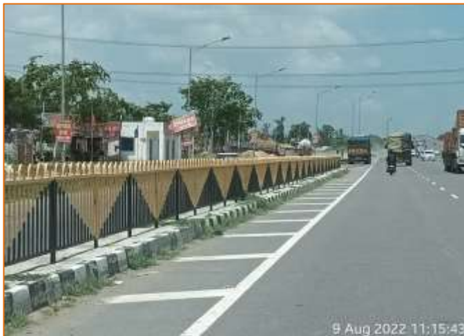
Pedestrian Guard Rail at km. 727+900
