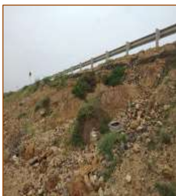
MJB at km. 474+405 (RHS)
