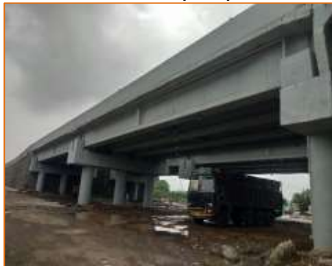
Side View of VUP (Limdi) at km. 23+120 (RHS)
