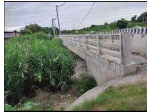
Minor Bridge at km. 75+009 (Structure View)
