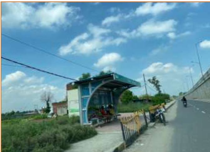
Bus Shelter at km. 775 + 900
