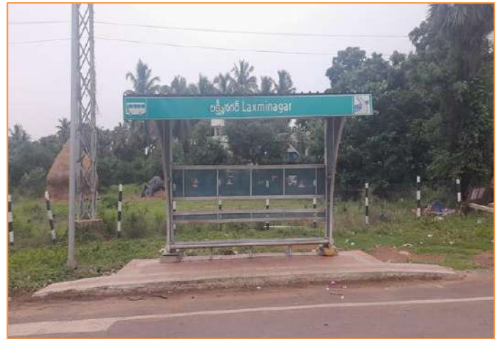
Bus Bay with Shelter at km. 56+140
