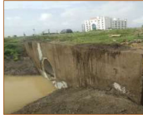
HPC at km. 490+350 (LHS)
