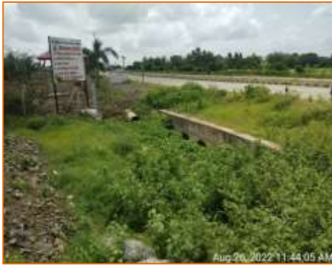
Pipe Culvert at km. 109.578 - RHS (Widening)
