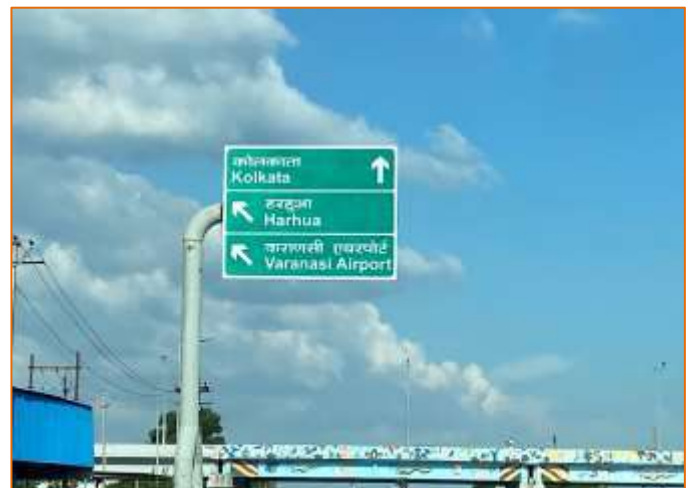
Cantilever Gantry Sign at km. 782+500
