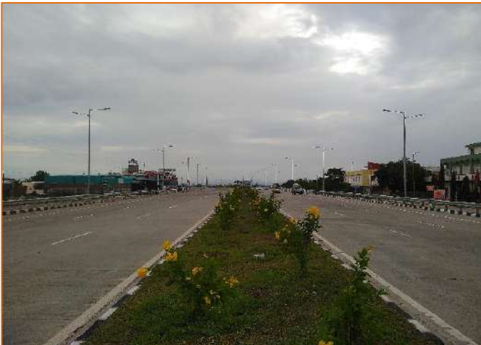
Pavement Condition at km. 285+750 (BHS)
