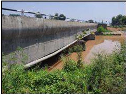
Minor Bridge at km. 48+323 (Existing Structure View)
