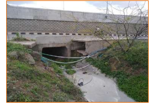
Box Culvert at km. 285+300
