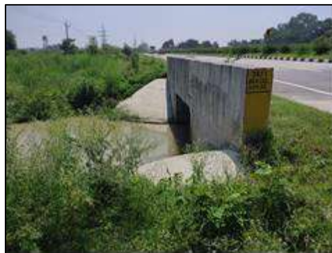
Box Culvert at km. 37+480
