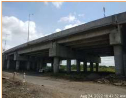
Side View of Flyover at km. 99.900 (LHS)
