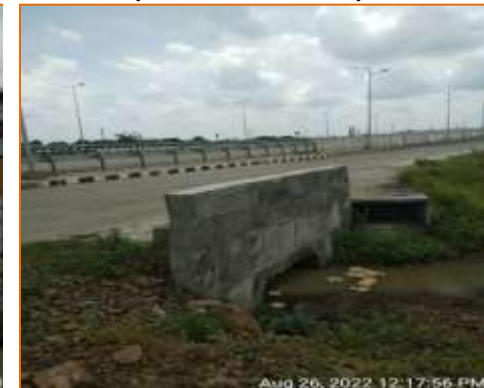
Box culvert at km. 133.524 - LHS (Reconstruction)
