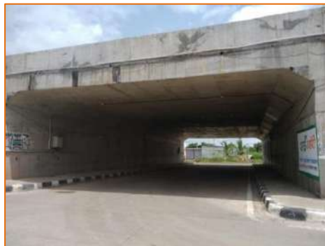
Light Vehicular Underpass at km. 276.900
