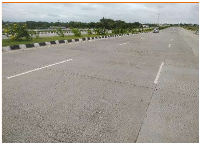
Road Markings at km. 306+500
