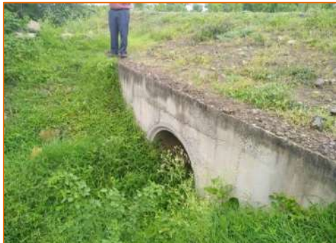
Pipe culvert at km. 311+550
