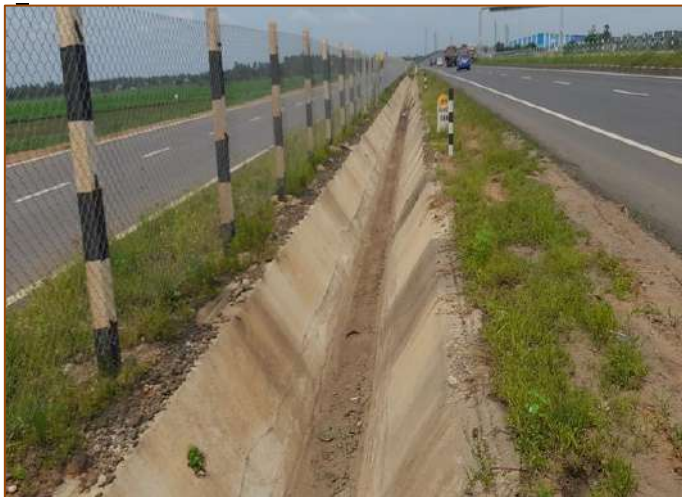
V Drain at km. 78+900
