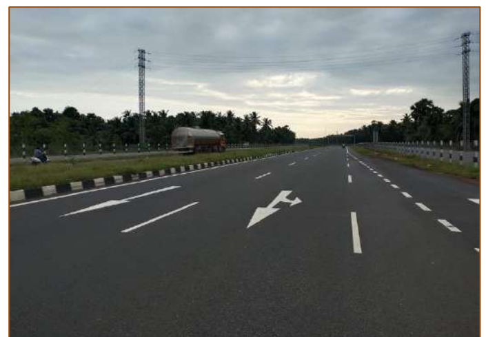
Road Markings at km. 56+760
