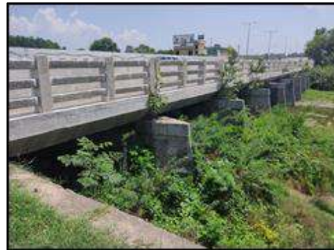
Major Bridge at km. 59+381 (Existing Structure View)
