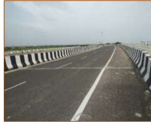
Wearing Coat of MJB at km. 395+255 (LHS)
