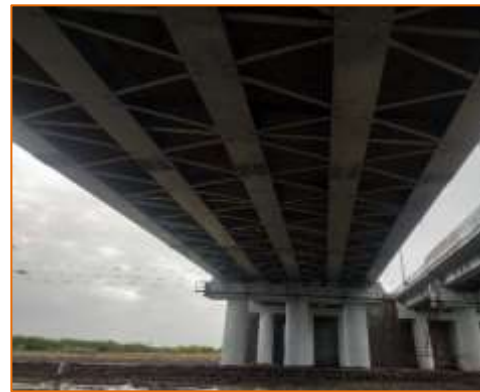
Bottom View of ROB's Girders at km. 0+527
