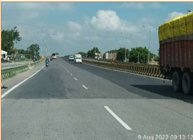
Road Marking to be done at km. 779+850
