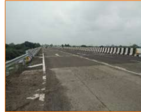
Wearing Coat of Major Bridge at km. 54+855 (RHS)
