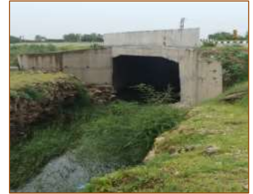
Minor Bridge at km. 385+350 (RHS) - Under COS
