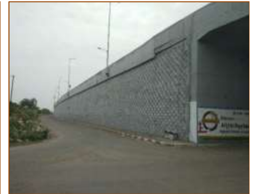
VUP at km. 396+865 (RHS) - A1 side
