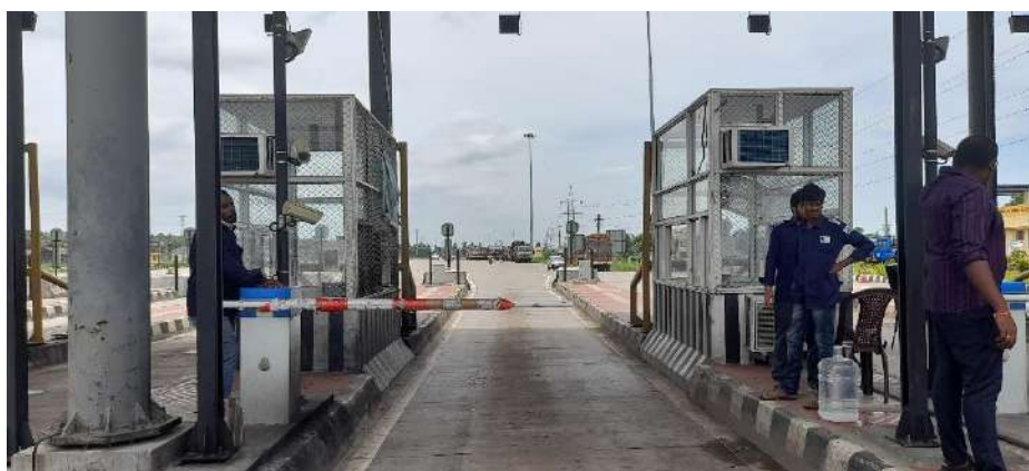
Figure 9-6 Automatic Lane Barrier
