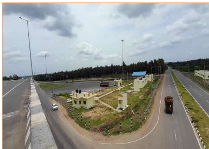
Rest Area at km. 66+800
