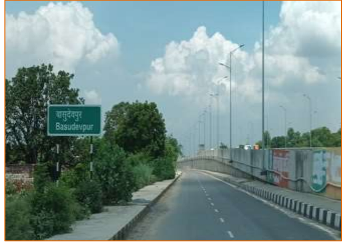
Drain at Service Road at km. 757+200
