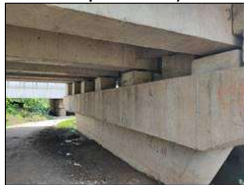
Minor Bridge at km. 71+174 (Substructure and Superstructure)
