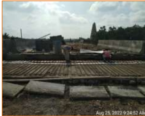
Approach slab work @ A2 side of Flyover is in progress at km. 136.857 (LHS)
