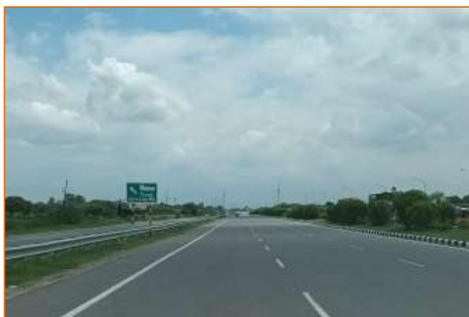
Truck Lay Bye at km. 727+900
