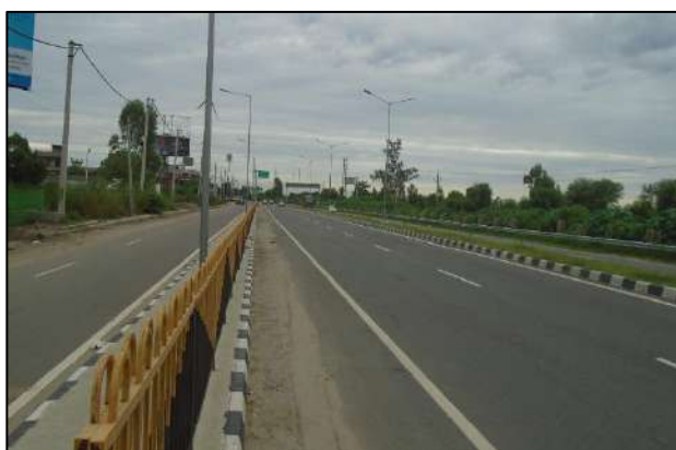
Approach to End of Project Road
