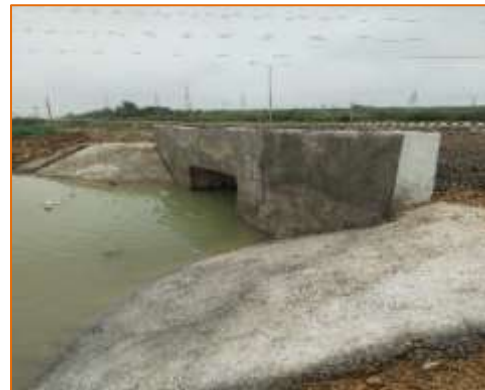
Box culvert at km. 11+950 (RHS)
