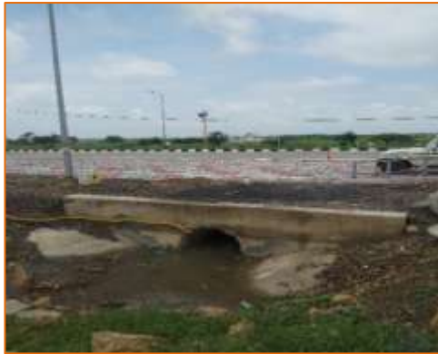
HPC at km. 5+800 (RHS)
