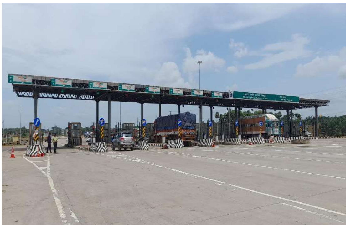
Figure 9-1 View of Toll Plaza (km. 53+700)
