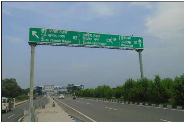
Overhead Gantry Sign Board at km. 8+400
