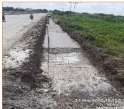
km. 133.300 WIP (RHS)
