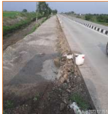
km. 46+000 single lane constructed
