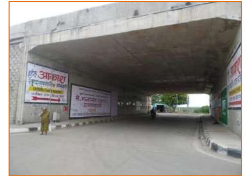
Light Vehicular Underpass at km. 283.650
