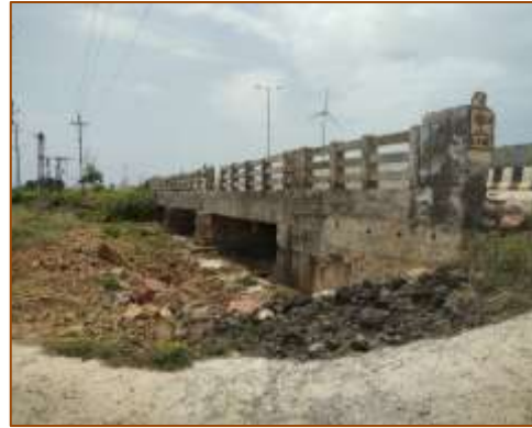
Side View of Minor Bridge at km. 449+894 (RHS) - Widening
