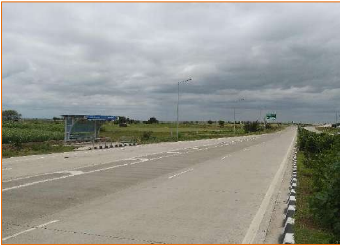
Bus Bay on service road at km. 305+800
