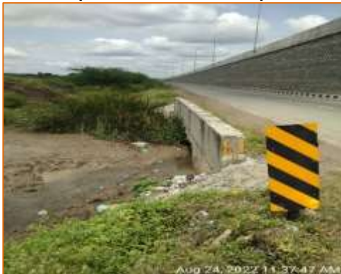
Box culvert at km. 103.850 - LHS (MCW & SR - New Construction)
