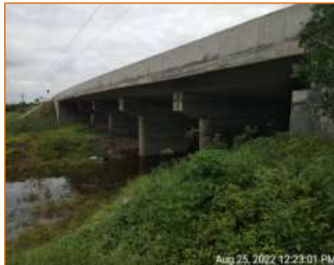
Side View of Minor Bridge at km. 124.337 (LHS)
