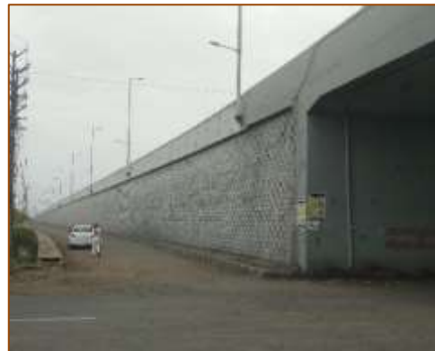
VUP at km. 400+681 (RHS) at A1 side
