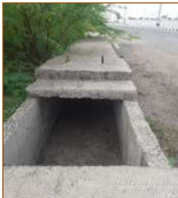
Built up drain from km. 489+000 to km. 490+000 (LHS)
