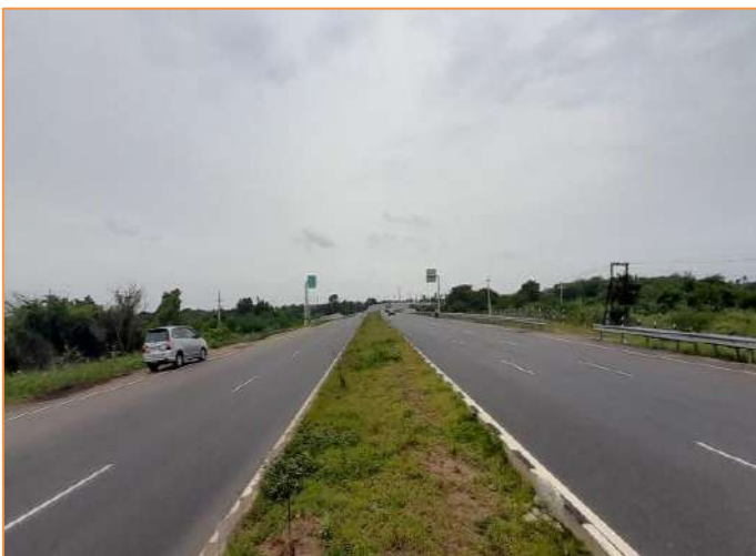
Pavement Condition at km. 55+100
