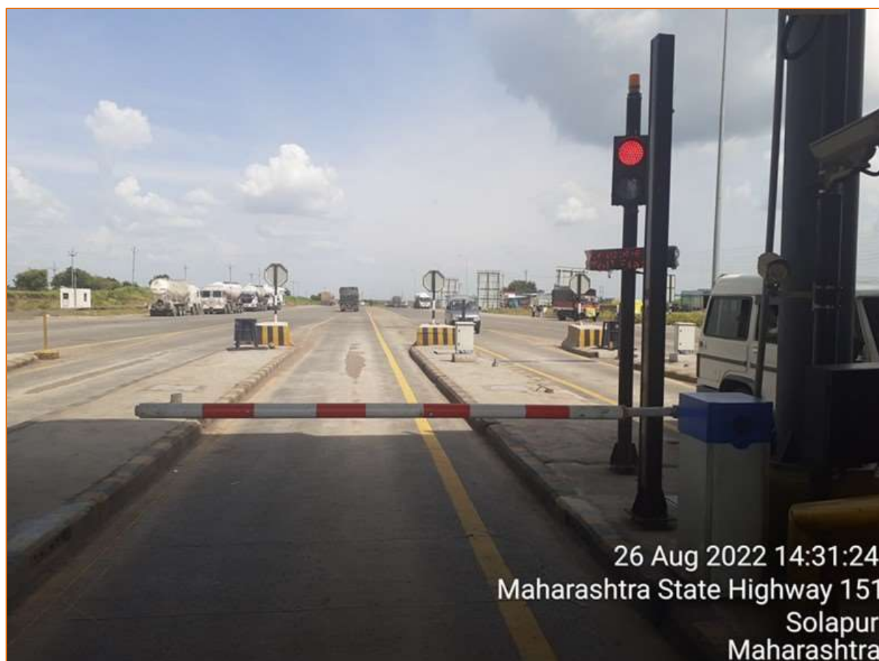
Figure 9-4 Automatic Lane Barrier
