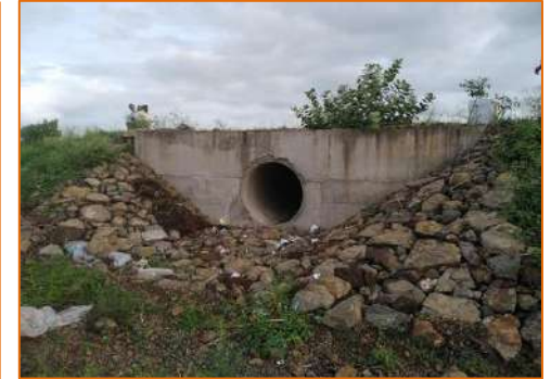
Pipe culvert at km. 310+423
