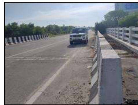
Minor Bridge at km. 71+727 (Top View)
