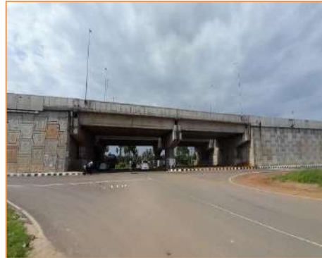
View of Flyover at km. 45+645
