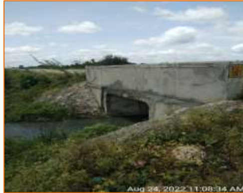
Box culvert at km. 101.823 - RHS (New Construction)
