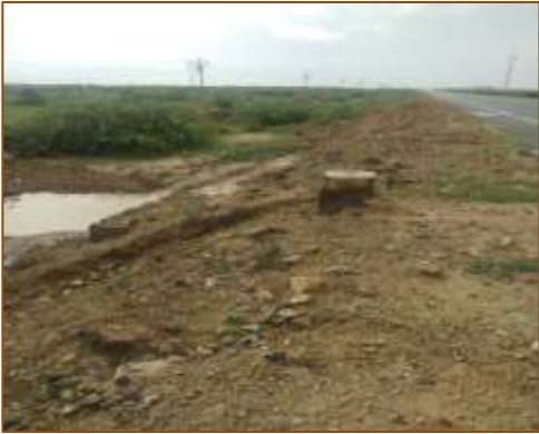
HPC at km. 487+054 (LHS)
