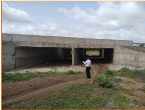
New Minor Bridge at km. 296.580
