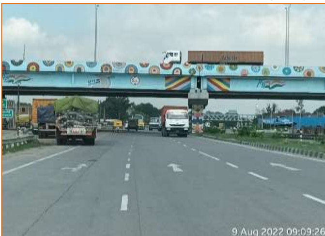
Pavement Condition at km. 782+500 (RHS)
