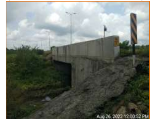
Box culvert at km. 105.290 - LHS (New Construction)
