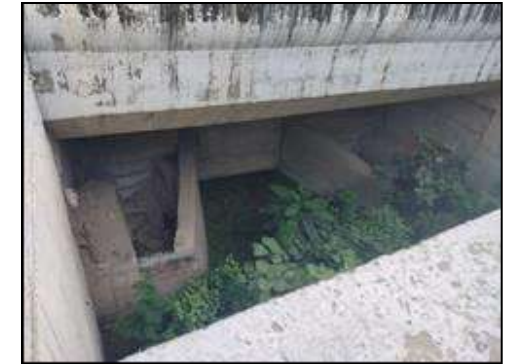
Minor Bridge at km. 69+815 (Existing Structure View)
