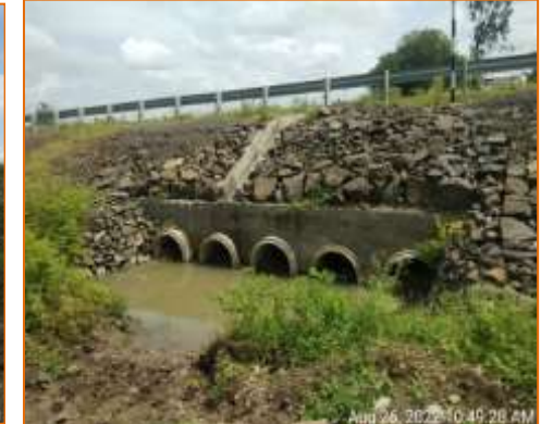
Pipe Culvert at km. 124.106-LHS (Widening)
