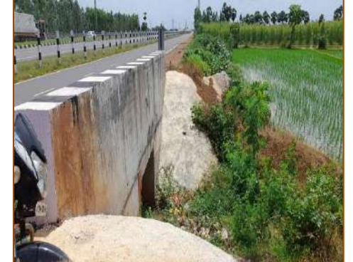
Box Culvert at km. 56+650
