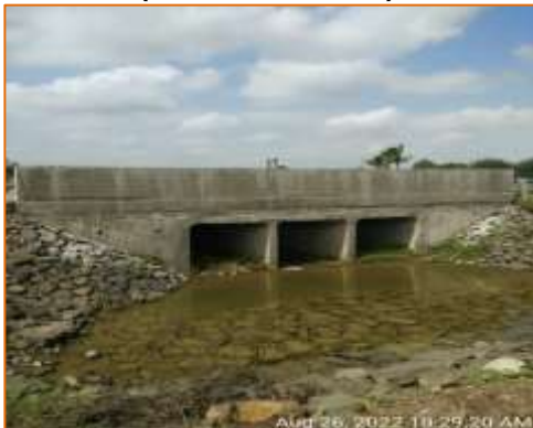
Box culvert at km. 128.229 - RHS (Reconstruction)
