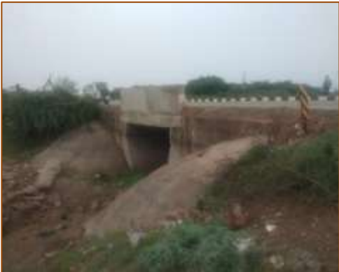
Slab culvert at km. 444+062 (LHS)
