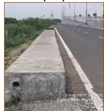
Built-up drain from km. 396+499 to km. 397+466 (RHS)
