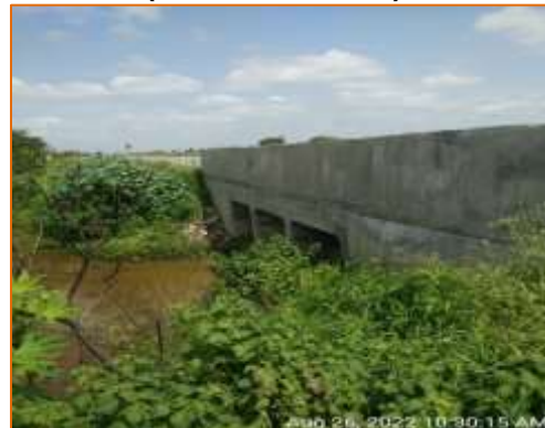
Box culvert at km. 128.229 - LHS (Reconstruction)
