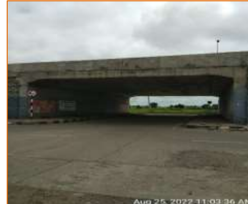
Side View of LVUP at km. 132.025 (LHS)
