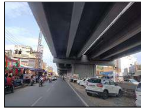
Elevated Structure at km. 25+319
