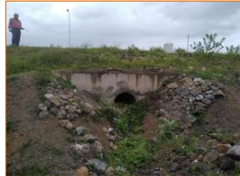
Pipe culvert at km. 318+657
