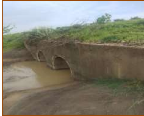
HPC at km. 487+054 (RHS)
