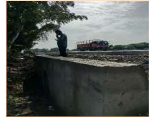
HPC at km. 32+520 (LHS)
