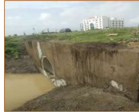
HPC at km. 490+350 (LHS)
