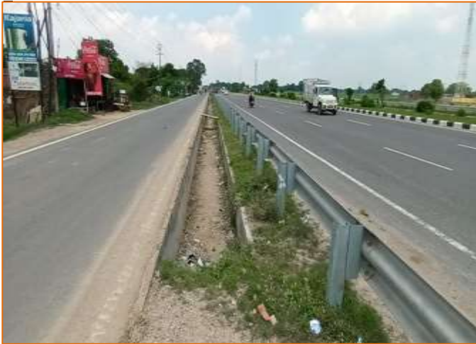
RCC Open Drain at km. 762+000
