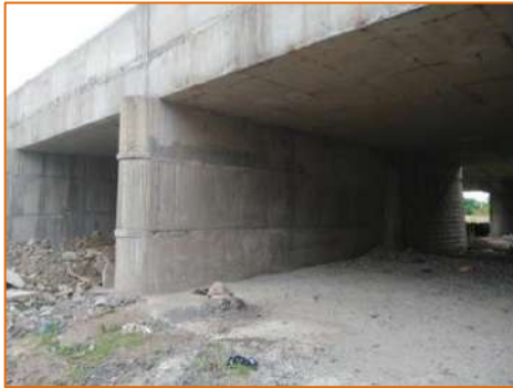
Widening of Existing Minor Bridge at km. 281.277
