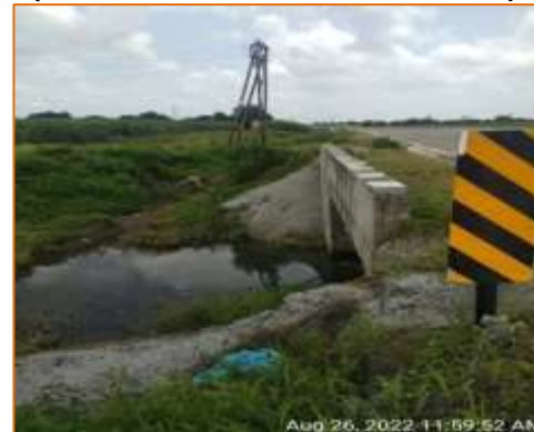
Box culvert at km. 105.290 - RHS (New Construction)
