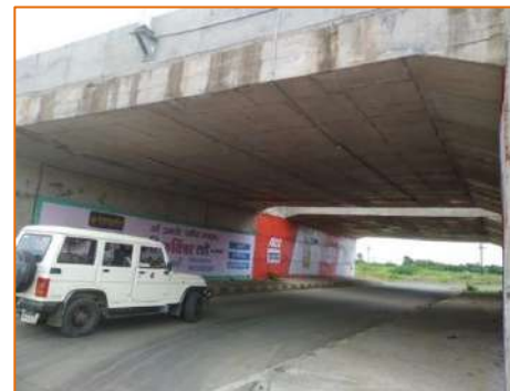
Light Vehicular Underpass at km. 320.900
