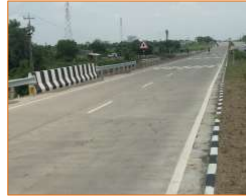
Wearing Coat of Minor Bridge at km. 64+660 (LHS)
