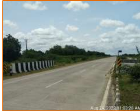
PQC of Minor Bridge at km. 101.260 (RHS)
