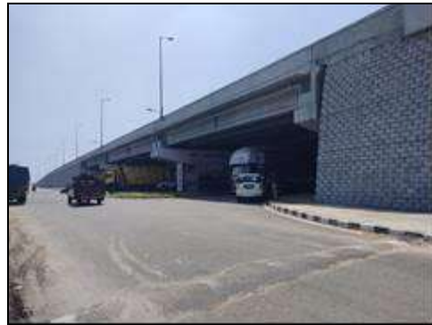
Flyover at km. 39+915
