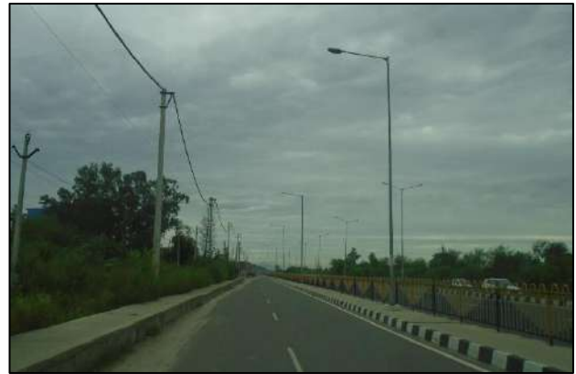
Street Lighting at Service Road
