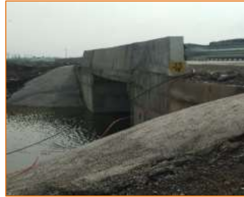
Side View of Minor Bridge at km. 34+400 (RHS)
