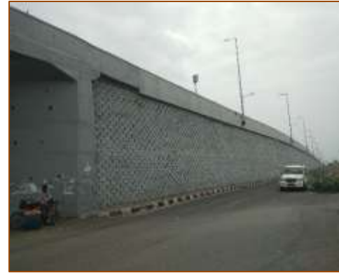
VUP at km. 397+096 (LHS) - Skew - A1 side
