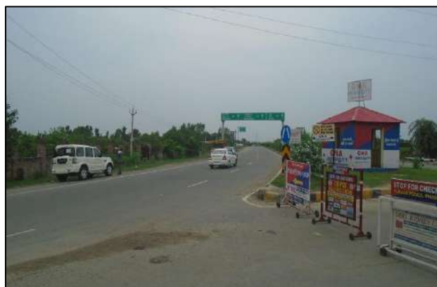
Start of Project Road - Left Carriageway
