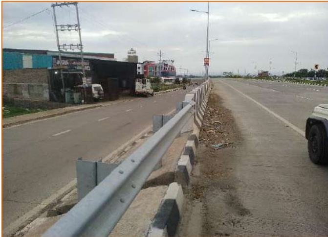
Crash Barrier at km. 285+650
