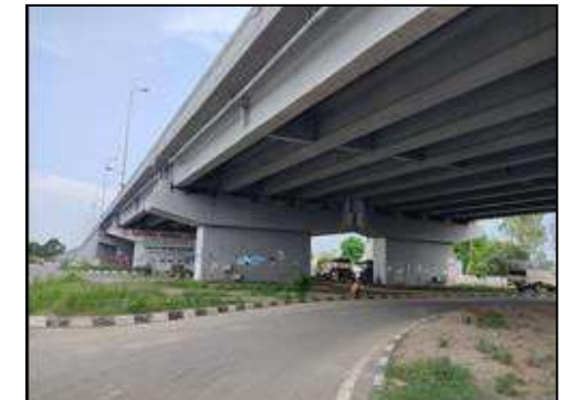
Flyover at km. 9+335
