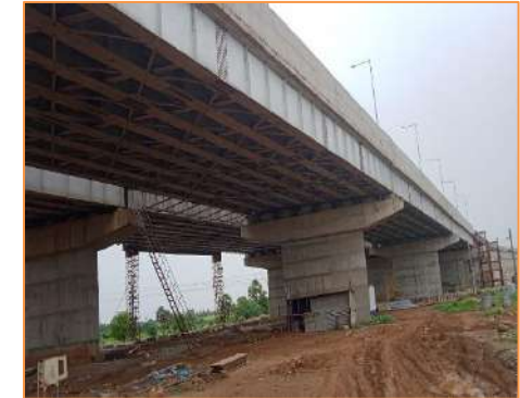
View of ROB at km. 18+677
