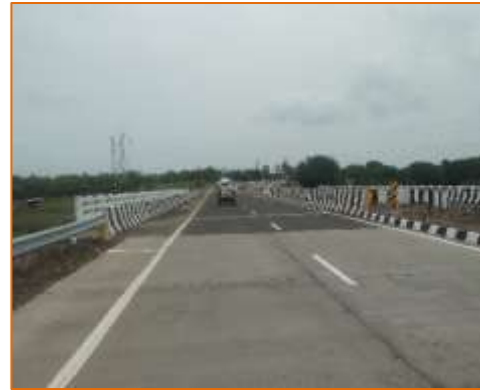
Wearing Coat of Major Bridge at km. 66+310 (LHS)
