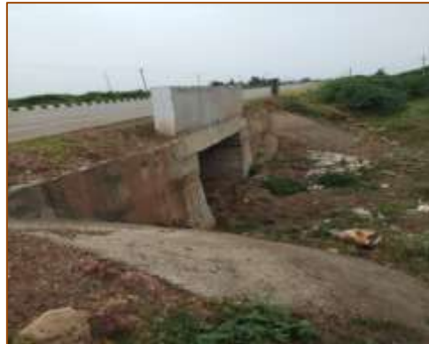
Slab culvert at km. 444+062 (RHS)
