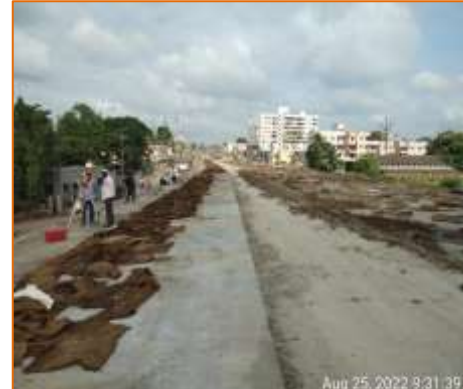
DLC & PQC of Flyover is in progress at km. 136.857 @ Solapur side (BHS)
