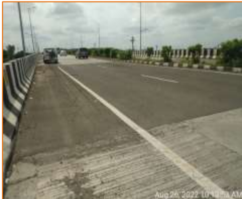
LVUP at km. 132.025 (RHS)
