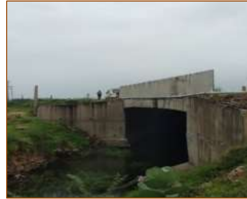
Minor Bridge at km. 385+350 (LHS) - Under COS
