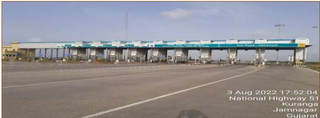
Figure 9-2 View of Okhamadi Toll Plaza
