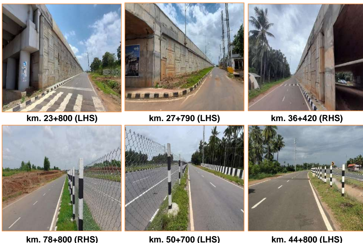
Figure 3-3 Photographs of Service Road
