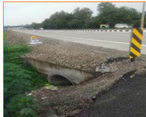
HPC at km. 66+010 (LHS)
