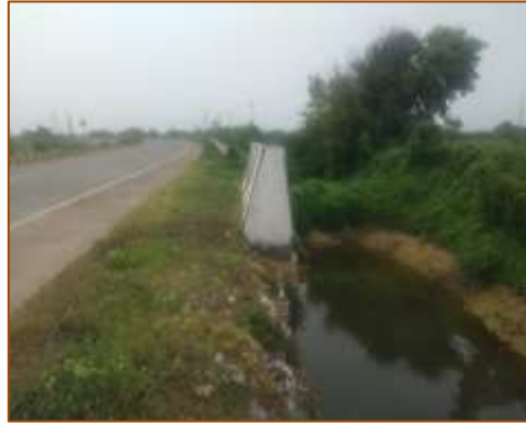
Slab culvert at km. 439+458 (RHS)
