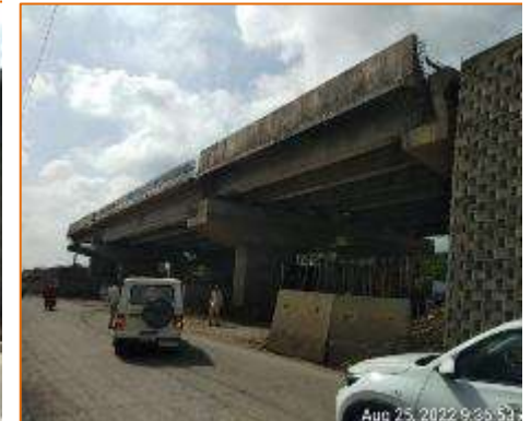
Side View of Flyover at km. 136.857 (RHS)
