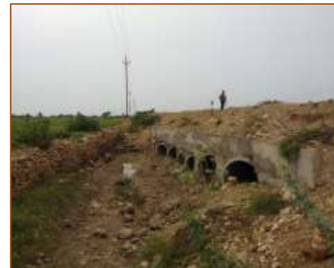
HPC at km. 456+200 (LHS)
