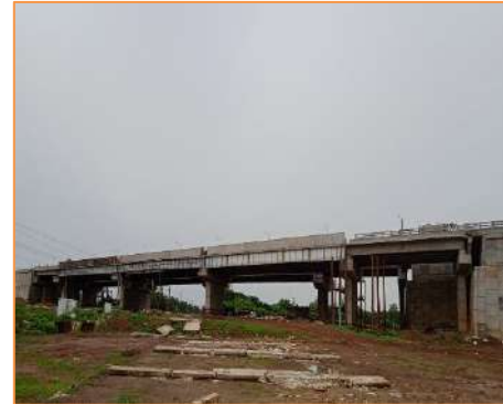
View of ROB at km. 18+677
